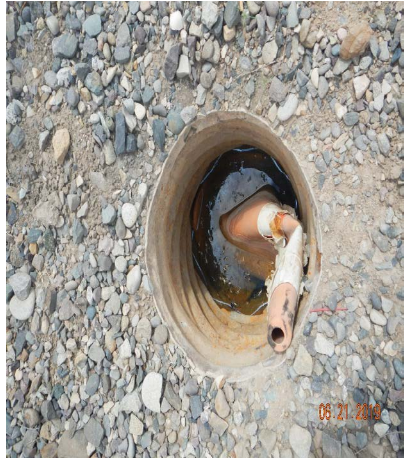
Photo#7: Open Rat Hole at Well API#077-09473.
