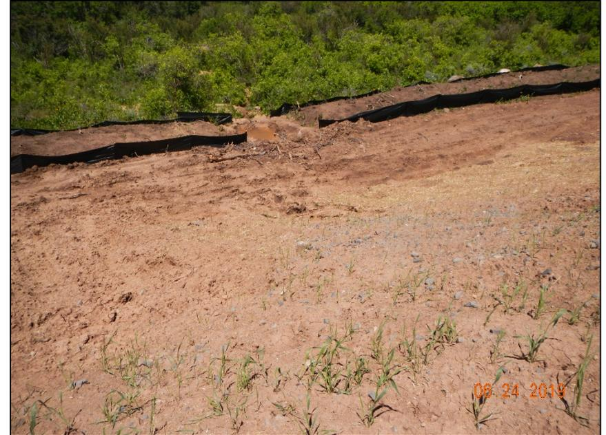
**Photo # 11 Photo of un-stabilized slope on West side of location**
