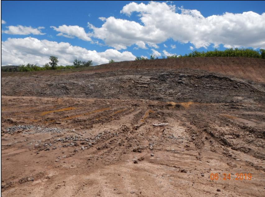
**Photo # 7 Photo Photo of Drill Cuttings on location not contained. Needs BMP**
