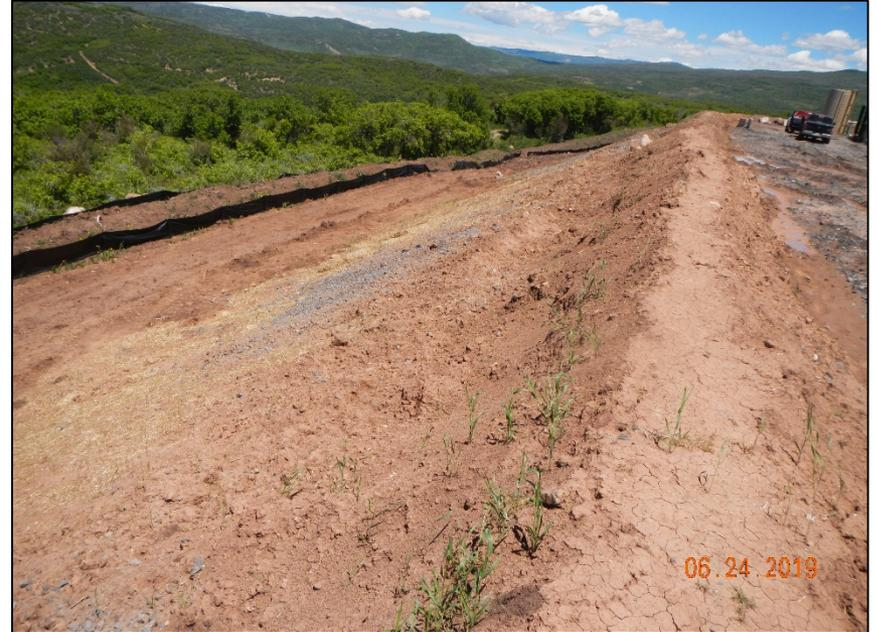
Photo # 13 Gravel over North side Berm
