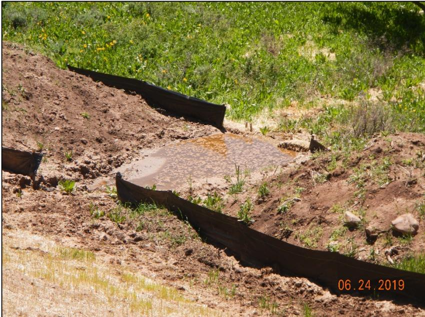
Photo # 9 Photo of Sediment Trap feeding retention pond needs maintenance.
