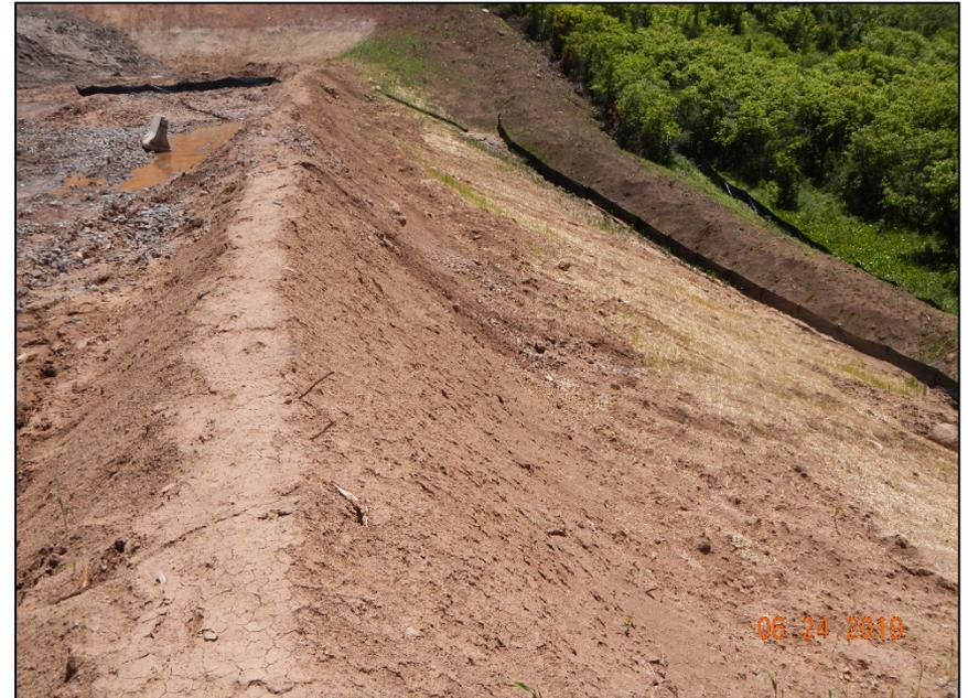
Photo #10 Photo of un-stabilized slope on West side of location
