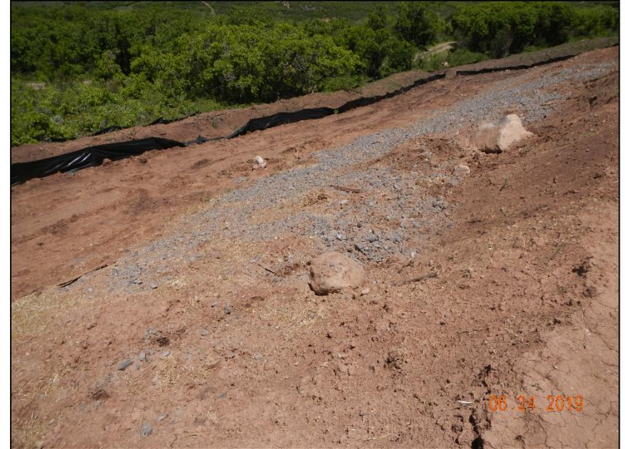
Photo #14 Gravel over North side Berm
