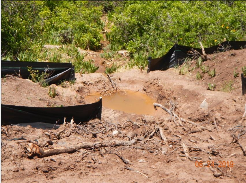
Photo # 12 Sediment trap needs maintenance.
