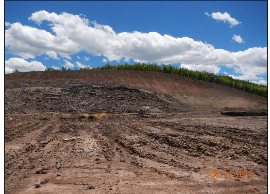
**Photo # 5 Photo of Drill Cuttings on location not contained.
