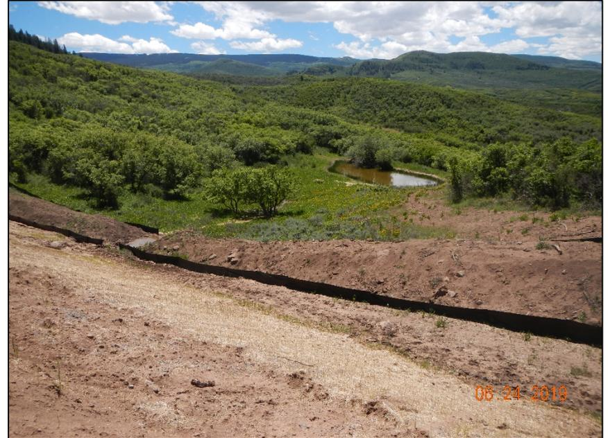
**Photo # 8 Photo of Sediment Trap feeding retention pond needs maintenance.**
