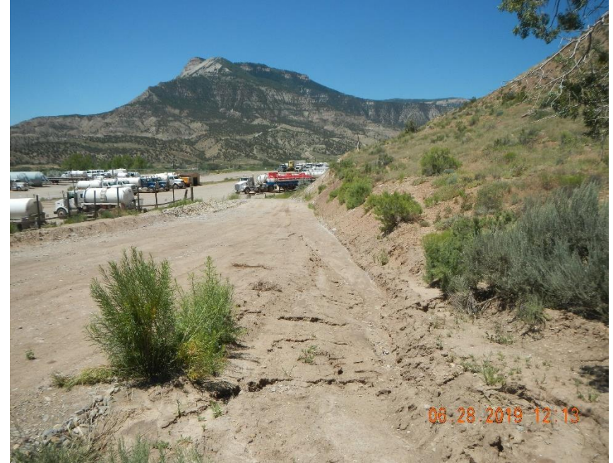
Sediment build up in road ditch along entrance access road.
