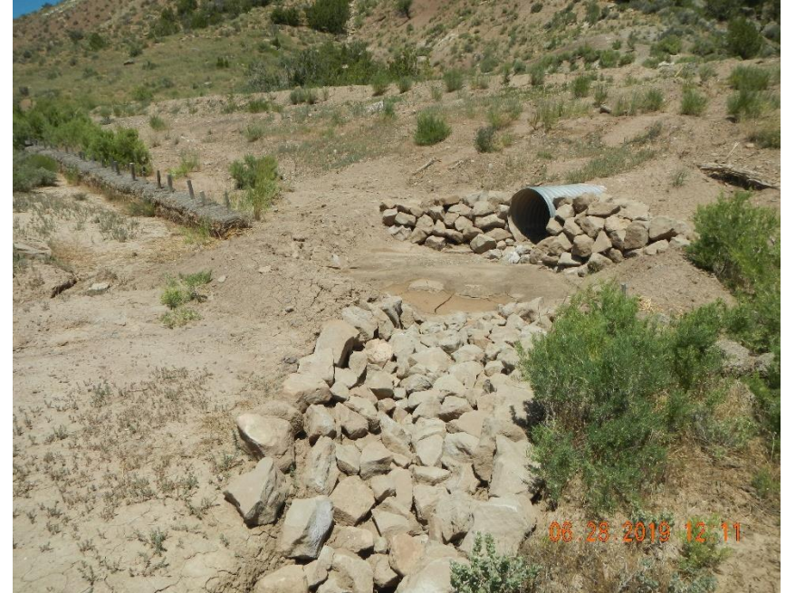
Culvert outlet basin maintained.
