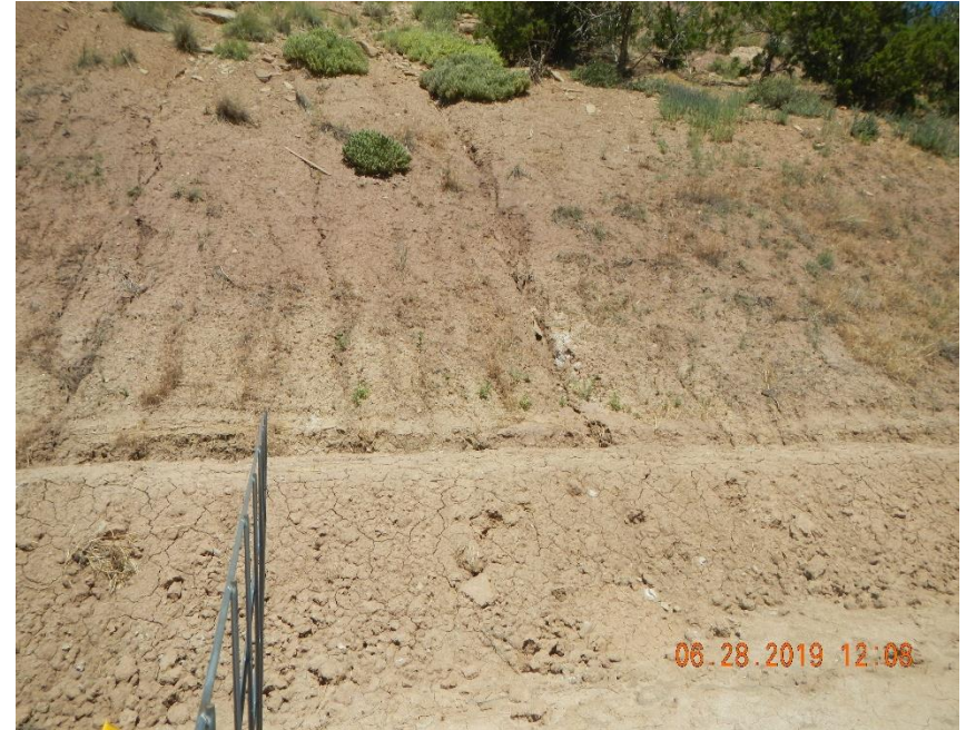
Washed out berm has been repaired.
