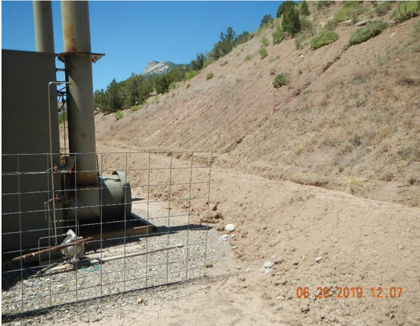
Washed out berm has been repaired.
