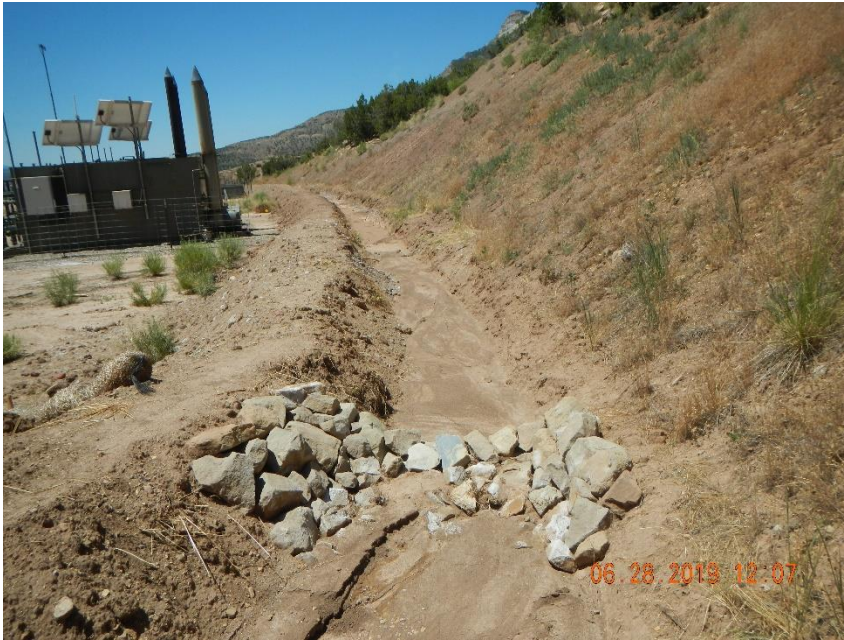
Ditch has been cleaned out and rip rap added.
