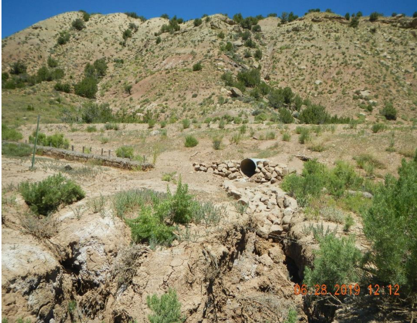
Erosion damage from culvert has not been repaired.
