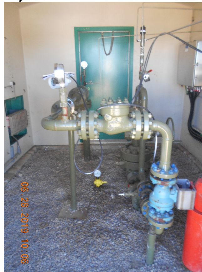
Injection Wellhead inside housing
