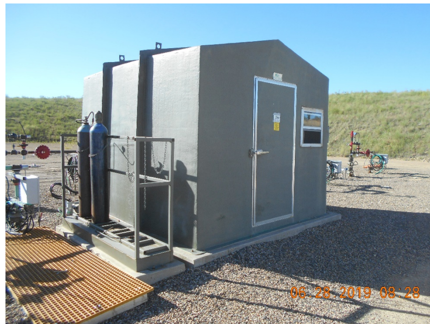
Injection wellhead housing
