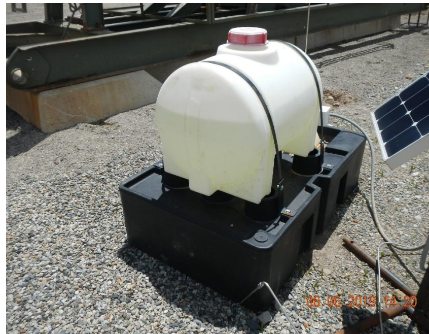
Unlabeled/unused chemical injection system.
