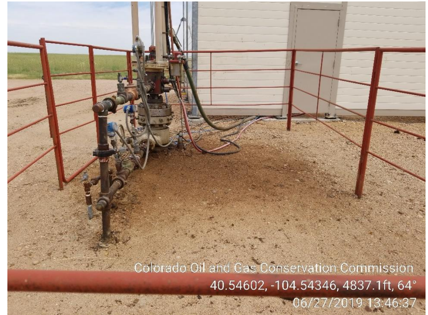
Photo 6 – Stained Soil at wellhead
