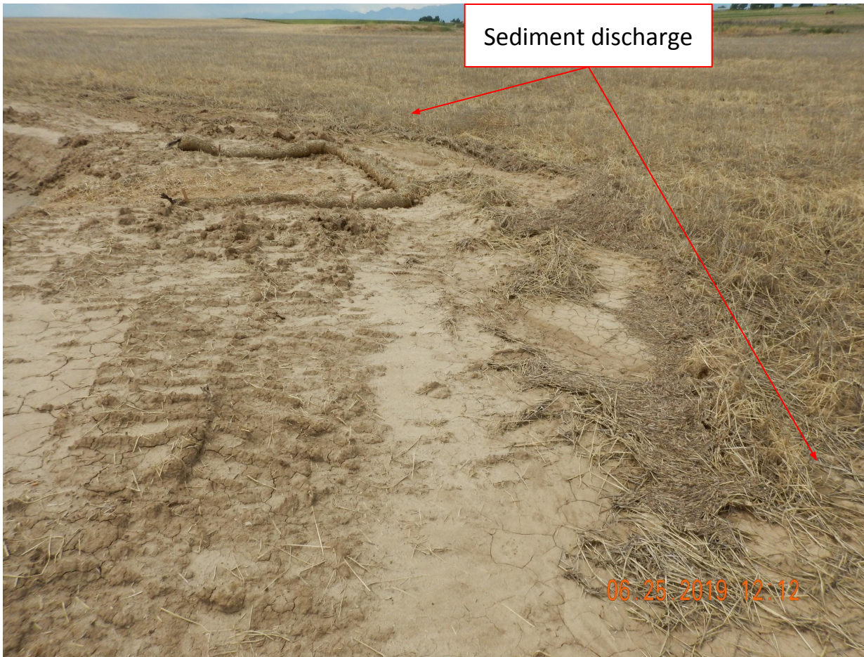
Photo 11. Close up photo taken from northwestern perimeter of location, facing West. Photo illustrates sediment discharge beyond the temporarily stabilized outlet (erosion control blanket).
