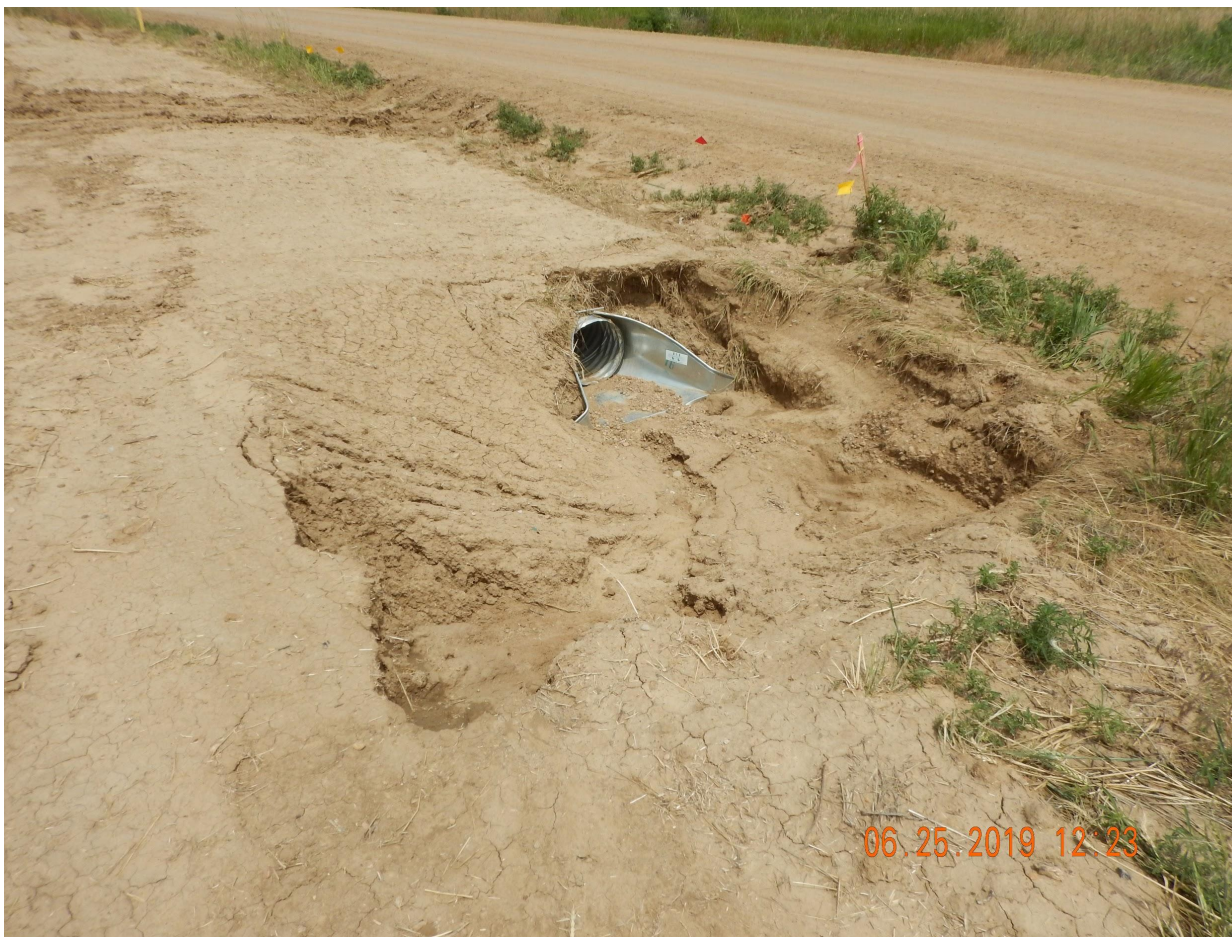
Photo 16. Photo taken from the north entrance of location, facing Northeast. Photo illustrates the Operator has failed to properly install the culvert with inlet protection, as gully erosion is observed at the inlet area.
