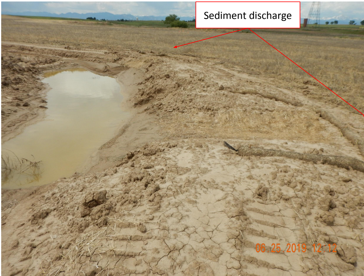
Photo 10. Photo taken from northwestern perimeter of location, facing West. Photo illustrates an improperly installed sediment trap. Operator has failed to install the sediment trap per good engineering practices and it has not been properly sized because sediment discharge was observed beyond the temporarily stabilized outlet (erosion control blanket)- see Photo 11.
