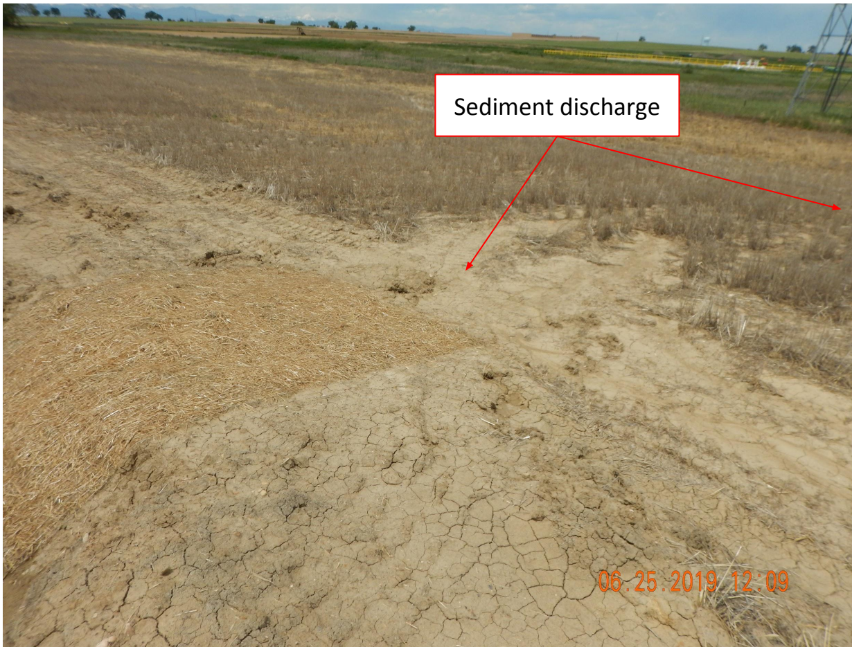
Photo 7. Photo taken from the northern perimeter of location, facing Northwest. Sediment discharge was observed beyond the temporary stabilized outlet (erosion control blanket). There was no observed sediment within the erosion control blanket which would imply it was installed after the discharge event.
