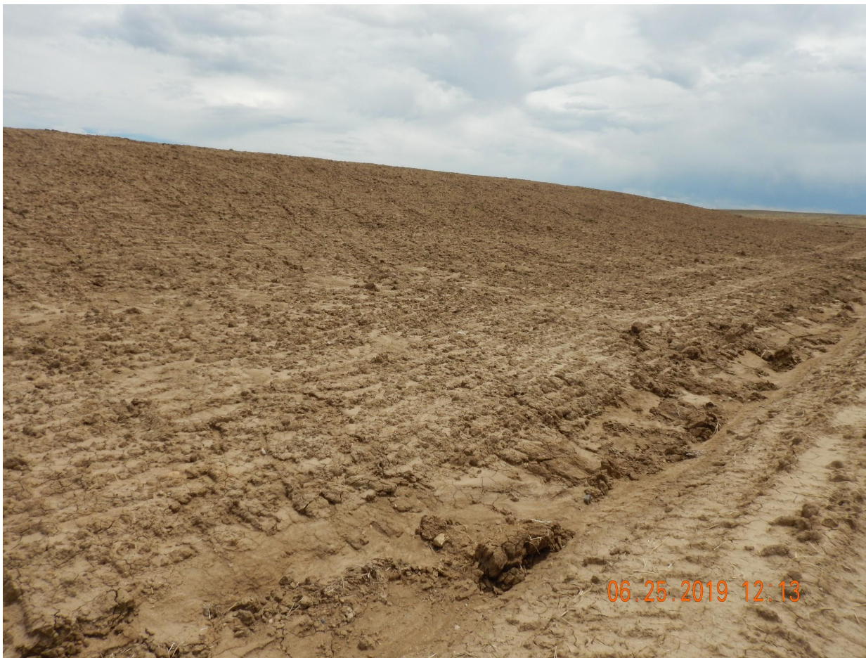
Photo 12. Photo taken from western perimeter of location, facing South. Photo illustrates the topsoil stockpile which has been temporarily stabilized but rill erosion was observed throughout.
