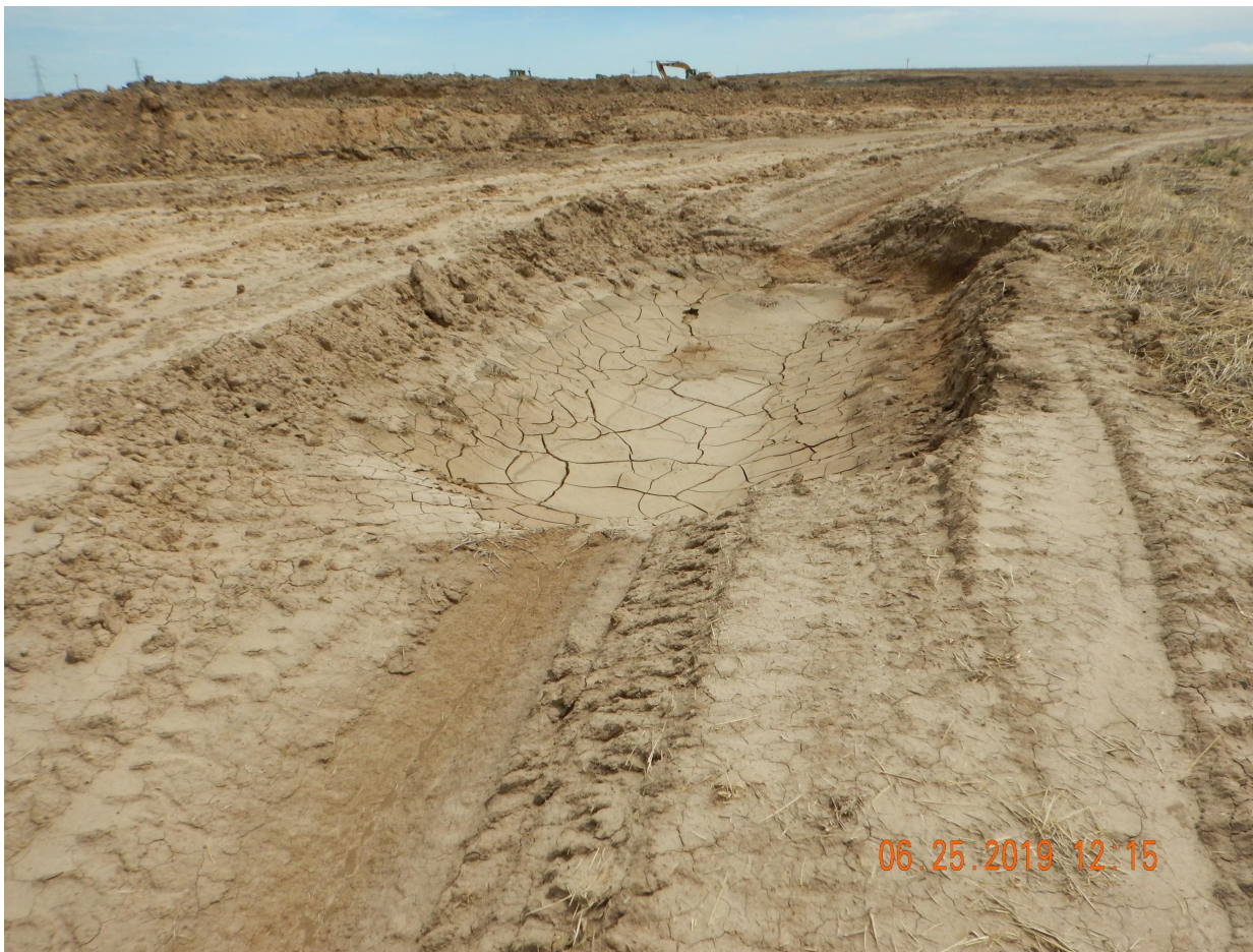
Photo 13. Photo taken from southwestern perimeter of location, facing East. Photo illustrates an improperly installed sediment trap. Operator has failed to install the sediment trap per good engineering practices, as the sediment trap itself appears to be eroding.
