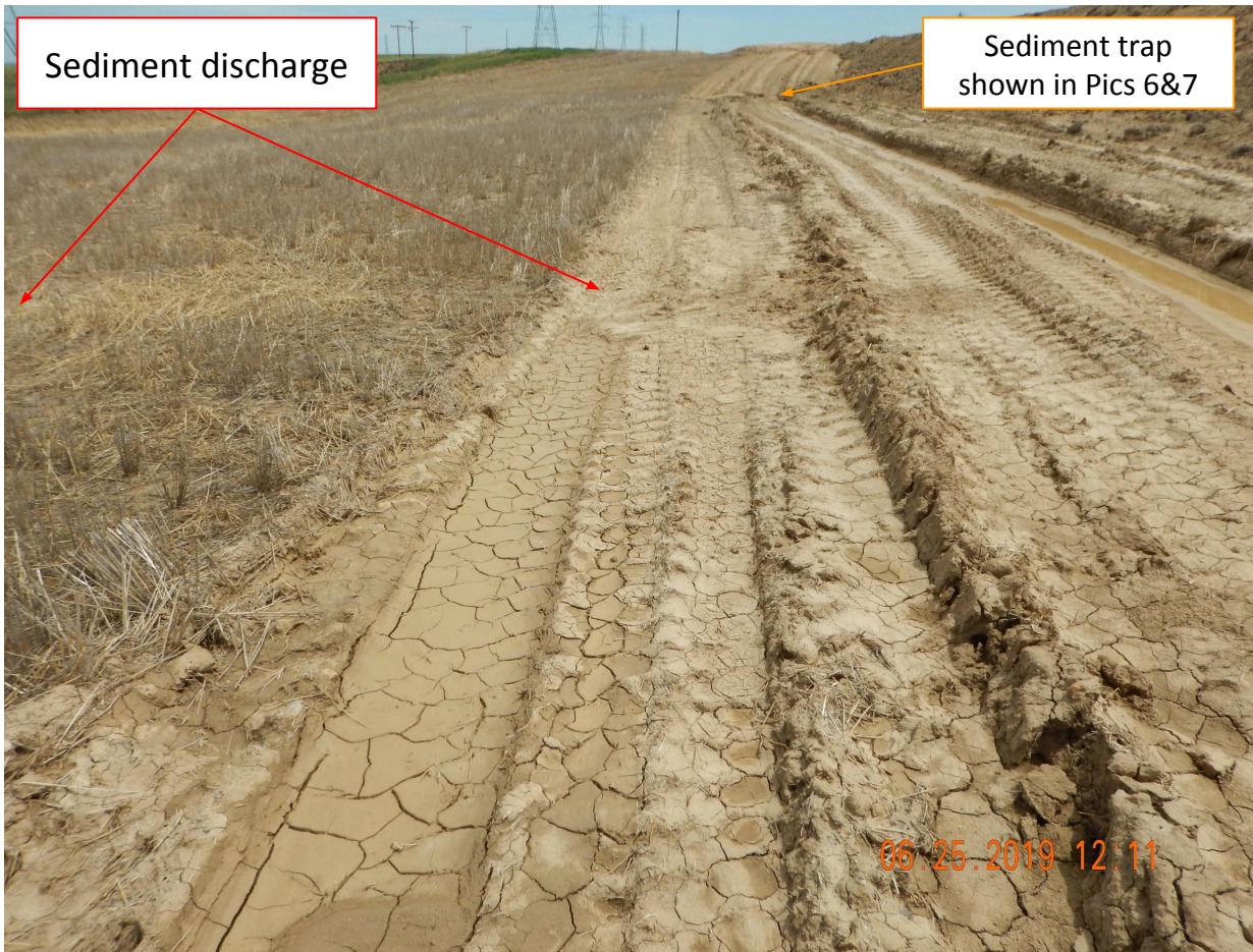
Photo 8. Photo taken from northwestern perimeter of location, facing East. Photo illustrates another point of discharge from location. Also, photo illustrates how the berm BMP has not been properly installed, as unconsolidated material has not been stabilized.
