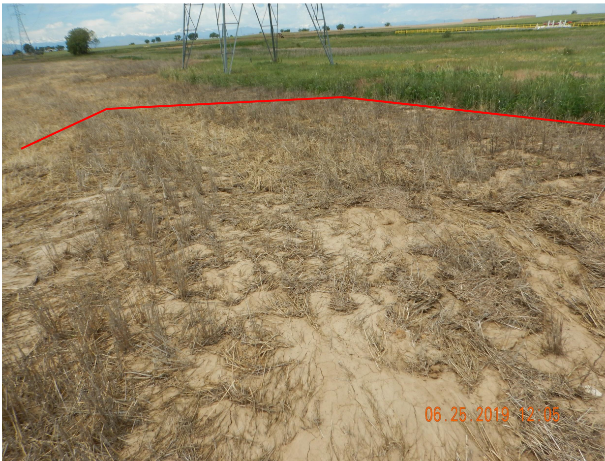
Photo 3. Photo taken from a portion of the northern discharge path, facing West. Photo illustrates sediment accumulation from stormwater erosion discharge from the location.
