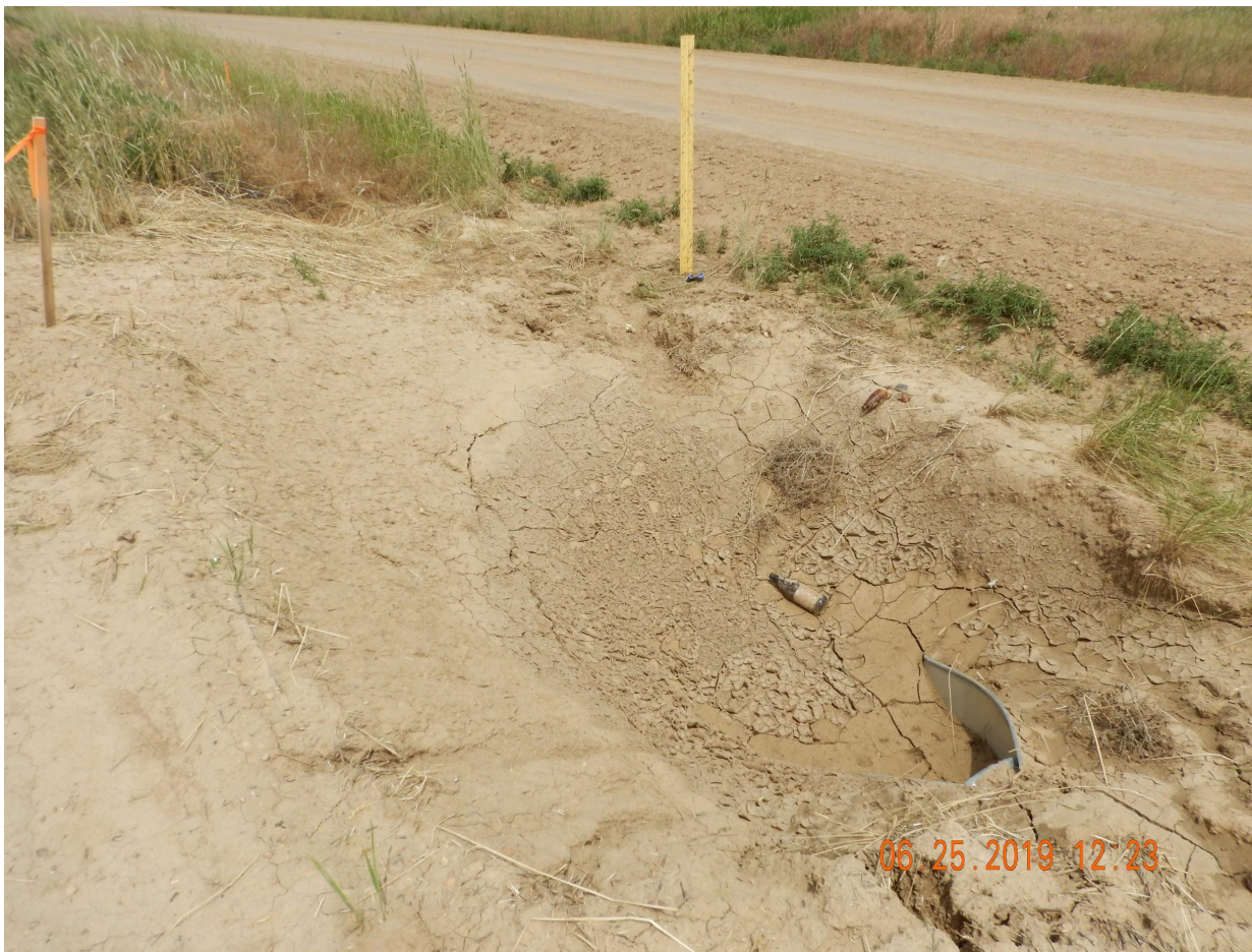
Photo 17. Photo taken from the north entrance of location, facing Northeast. Photo illustrates the Operator has failed to properly install the culvert with outlet protection, as sediment accumulation was observed at the outlet area.
