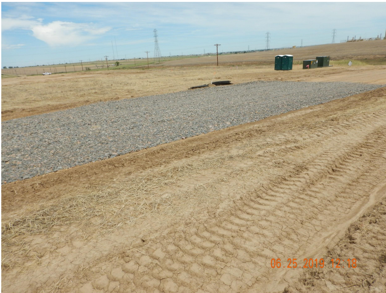
Photo 15. Photo taken from the southern entrance of location, facing Northeast. Operator has installed a vehicle tracking device BMP and it appears to be in proper functioning condition at the time of this inspection.
