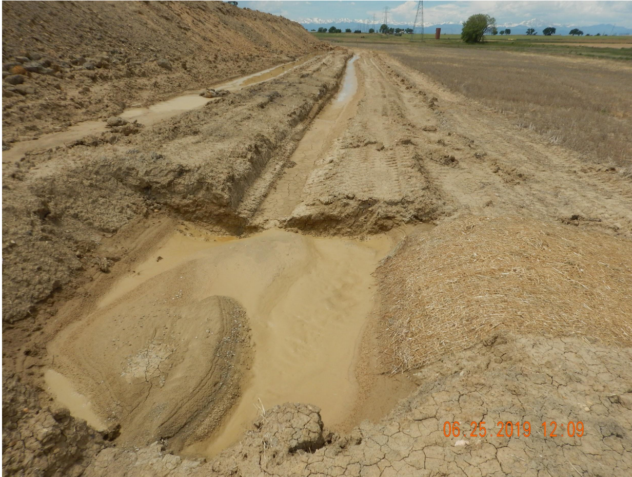
Photo 6. Photo taken from the northern perimeter of location, facing West. Photo illustrates an improperly installed sediment trap. Operator has failed to install the sediment trap per good engineering practices and it doesn't appear to be properly sized as sediment accumulation has almost filled it up. Based off my observations, the Operator installed this sediment trap after sediment had already discharged from location- see Photo 7.
