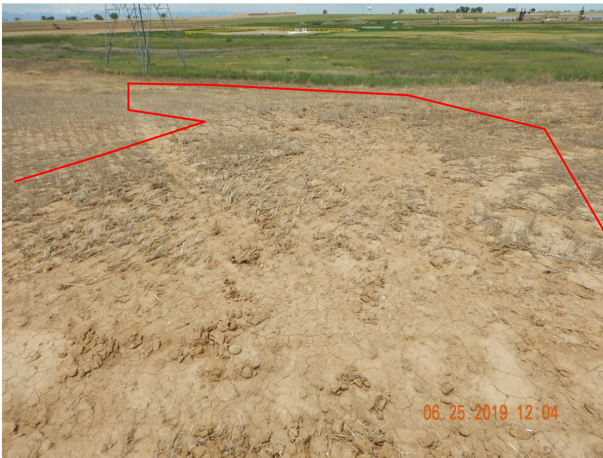
Photo 2. Photo taken from the discharge point along the northeastern perimeter of location, facing North. Photo illustrates wheat stubble that has been laid over due to stormwater erosion discharge from location.
