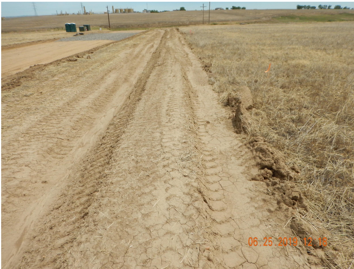
Photo 14. Photo taken from southern perimeter of location, facing East. Photo illustrates an improperly installed berm BMP, as unconsolidated material has not been stabilized.
