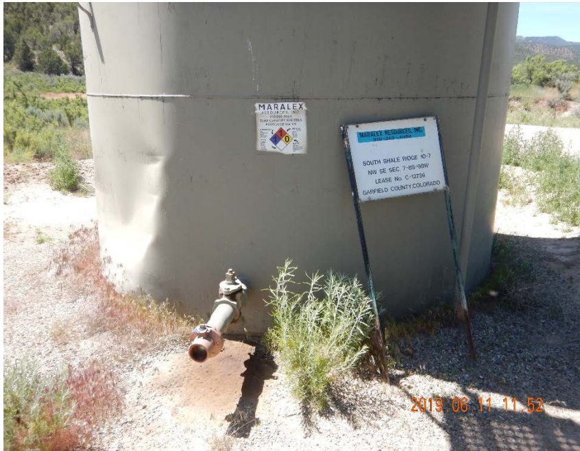
Photo #1 – Facility sign located at tank battery. Note accumulation of oil-stained soil beneath truck loadout and uncontrolled weeds in bermed area.
