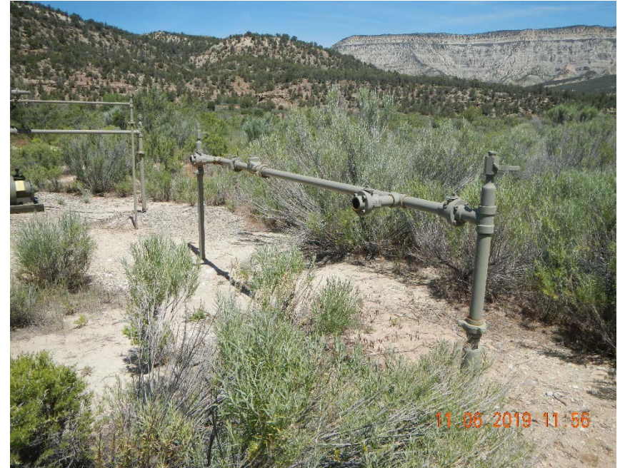
Photo #6 – Uncapped, unmarked flowline manifold west of pump jack. Note uncontrolled weeds in this location.
