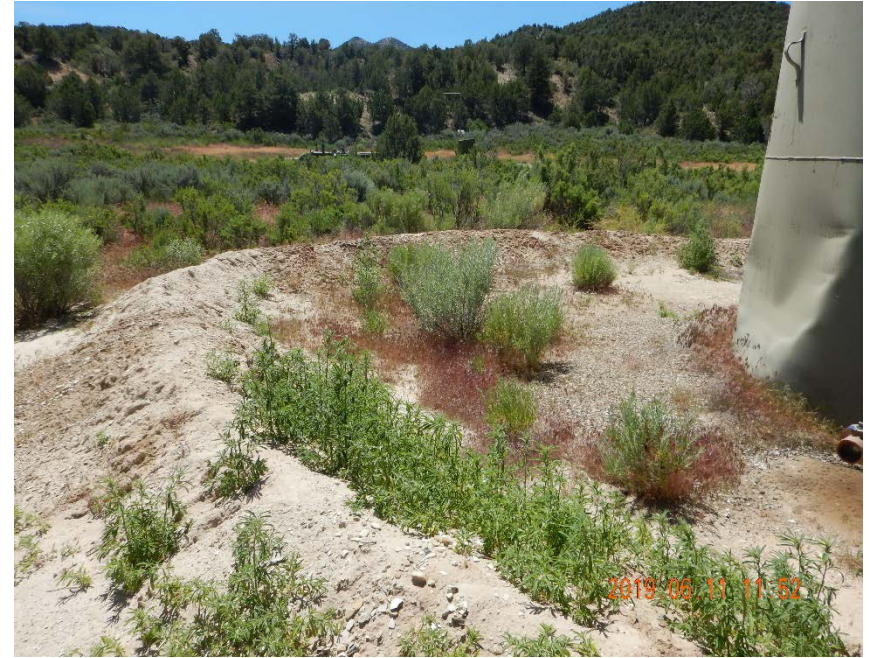
Photo #2 – Uncontrolled weeds and eroded berms at tank battery.
