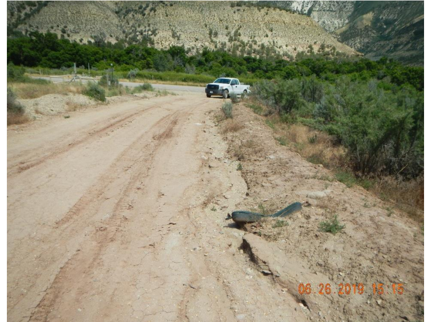
Washing of access road ditch
