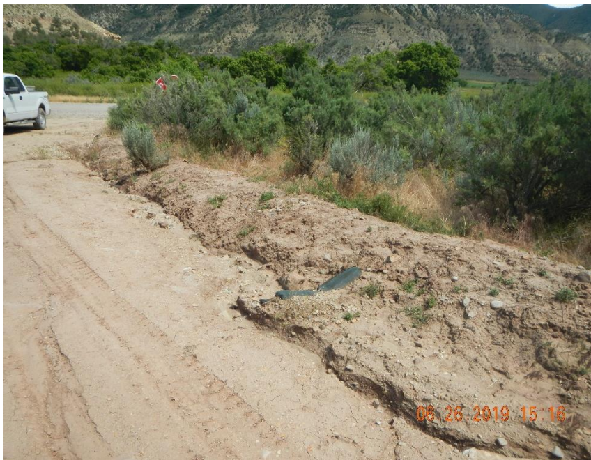
Washing of access road ditch
