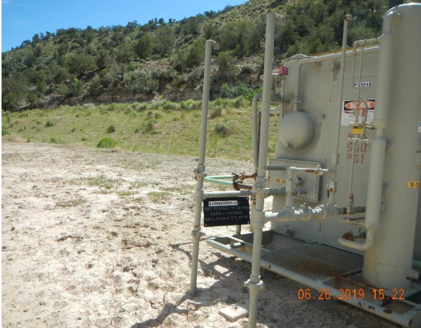
Separator and dehydrator unit combo
