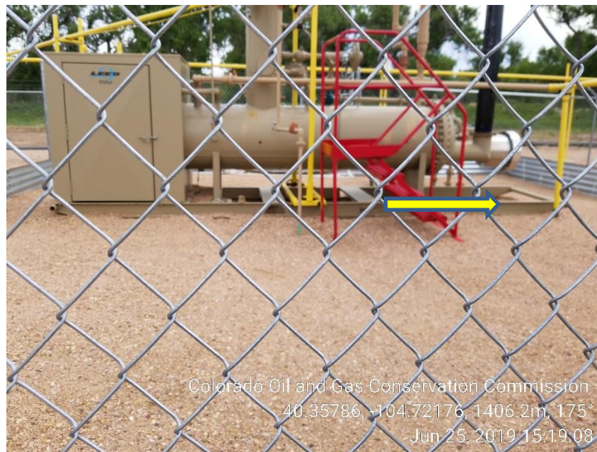
Photo 5: Separator NOT anchored
