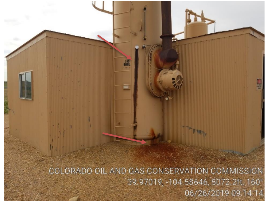
Pic 2, possible leak, stained soil
