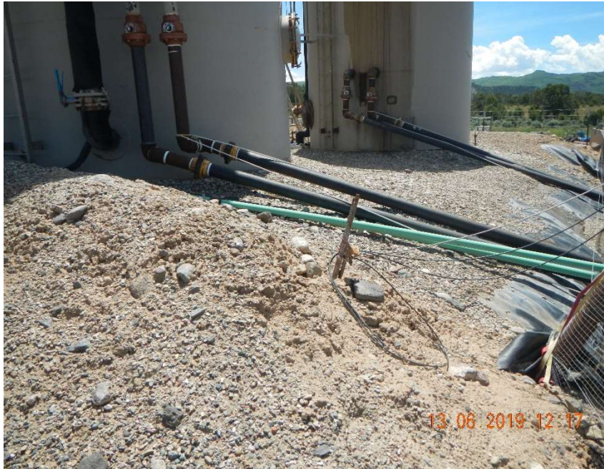
Photo #5 – View of the eroding earthen berm around the tank battery and the stained Steel AST tank.
