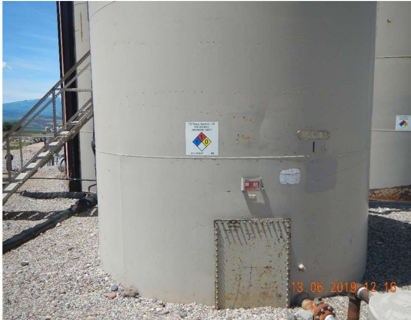
Photo #7 - Steel AST tank lacking tank capacity information.
