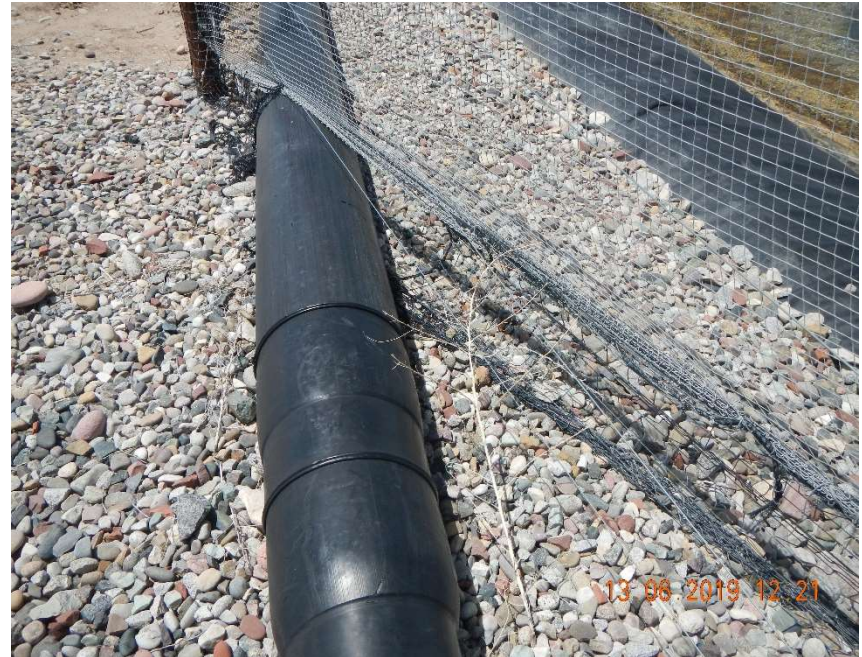
Photo #10 – Gaps (6-8 inches) in netting/fencing at poly pipe penetrations.
