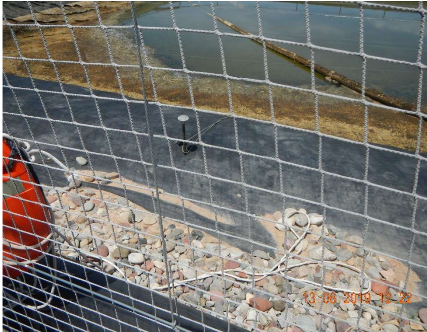
Photo #9 – View of the pit looking north with sediment in the pit bottom and a rebar stake that has been driven through the pit liner. Condensate was also observed within the pit.
