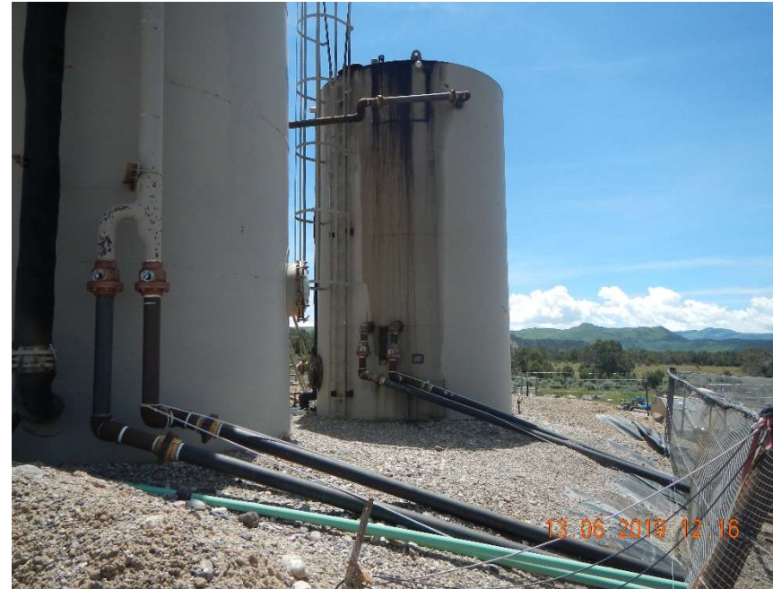
Photo #6 – Steel AST tank with staining.
