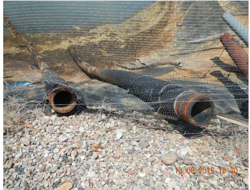
Photo #8 – Uncapped poly pipes leading into the pit.
