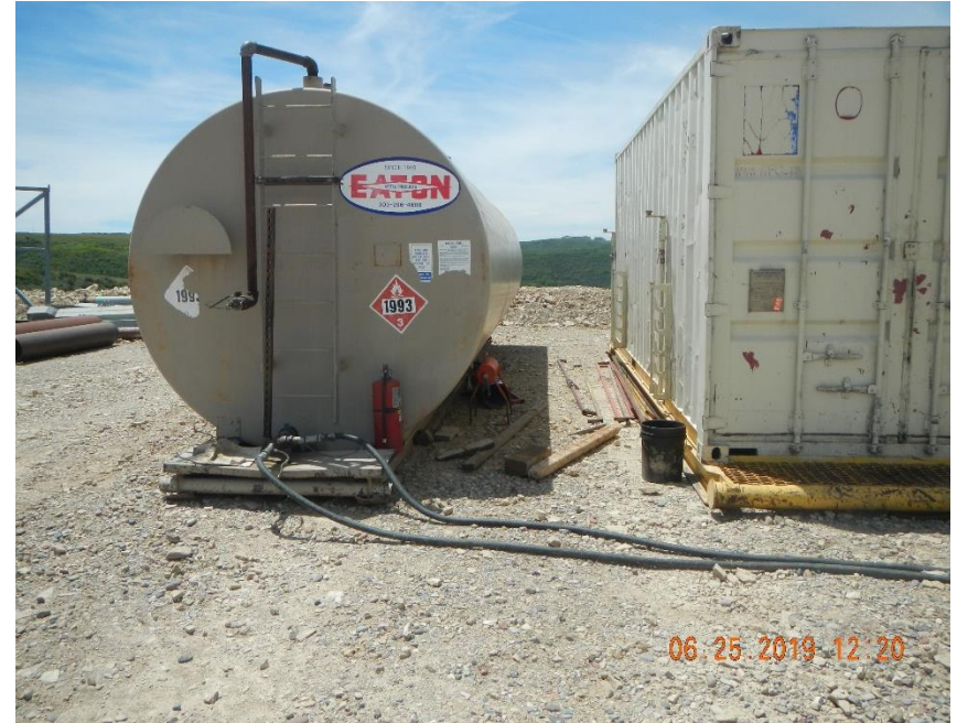
Unlabeled 5 gallon bucket by diesel tank has no secondary containment..
