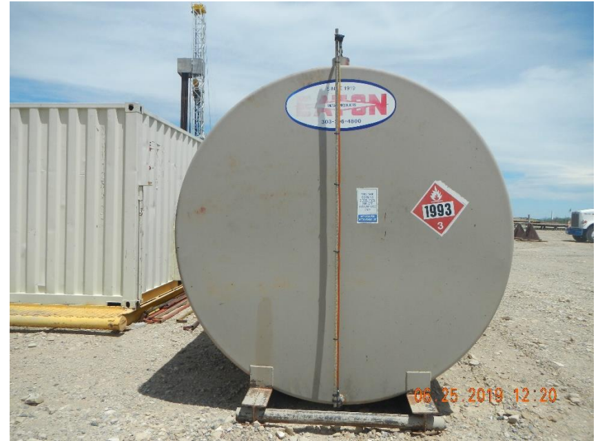
Diesel tank missing volume. Diesel tank with out 110 % containment.
