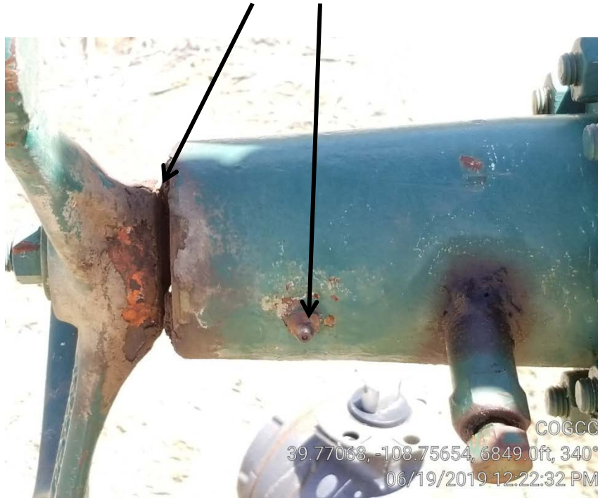
Photo 2. Gas leaks.
