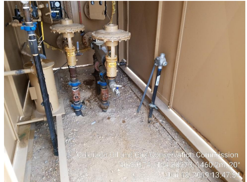
Photo 8: Stained soil in separator house
