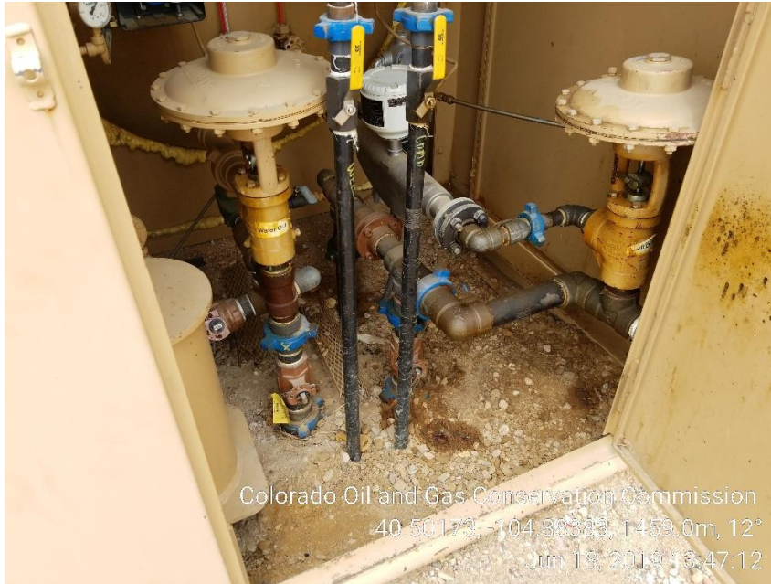
Photo 5: Stained soil in separator house
