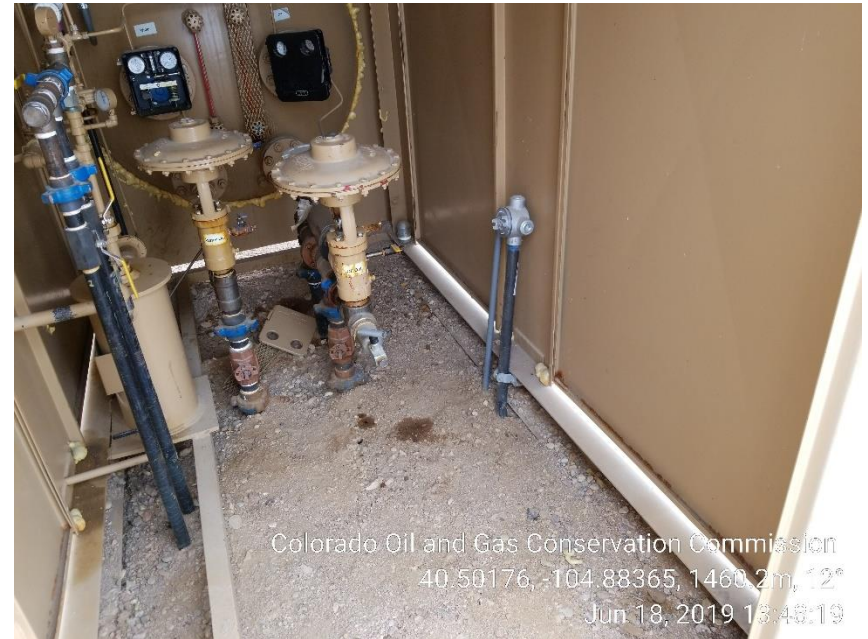
Photo 10: Stained soil in separator house
