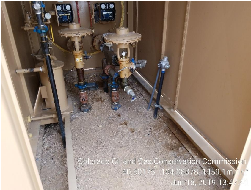
Photo 7: Stained soil in separator house
