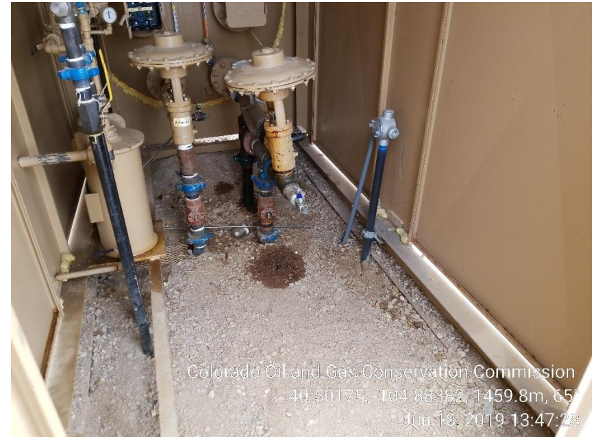
Photo 6: Stained soil in separator house
