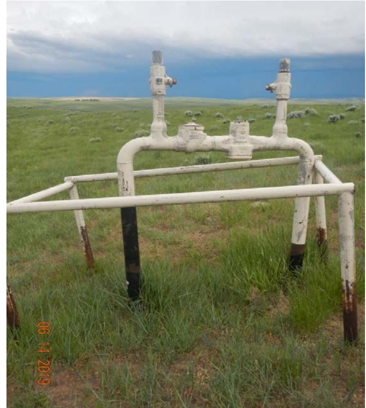
Photo#3: Close up of riser remaining on Location.
