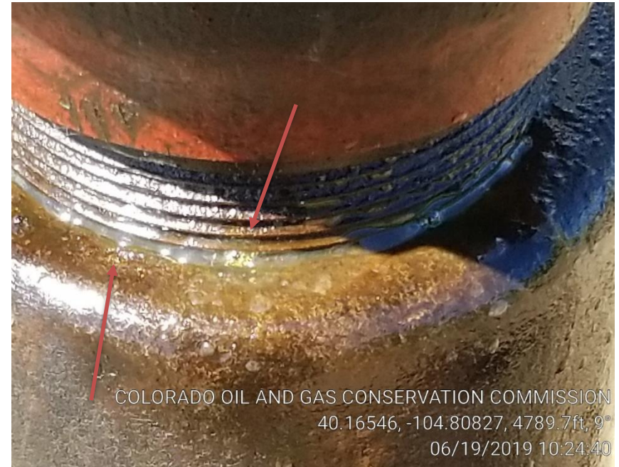
Pic 2 bubbles coming out of wellhead
