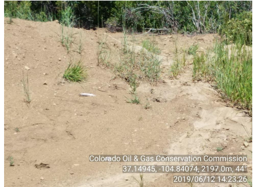
PHOTO 4: SEDIMENT TRAP JUST EAST OF ENTRANCE OF LOCAITON IS FULL W/ SEDIMENT AND IS ALLOWING STORM WATER TO CARRY SEDIMENT PAST BMP'S. CLEAN AND MAINTAIN SEDIMENT TRAP IN ACCORDANCE WITH 1002 SERIES STORMWATER RULES. CA DATE 7/12/19.
