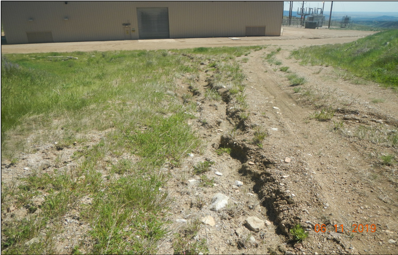
Photo 5. Facing down the access road. There is an erosion channel that has developed.
