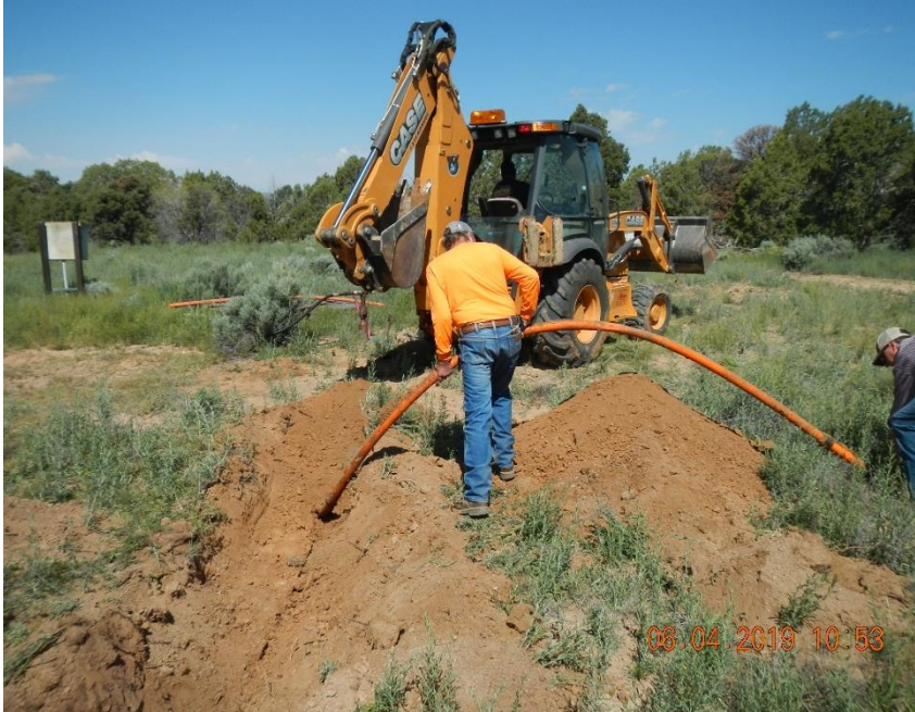
Moving poly pipe from wellhead connected to stand pipe.
