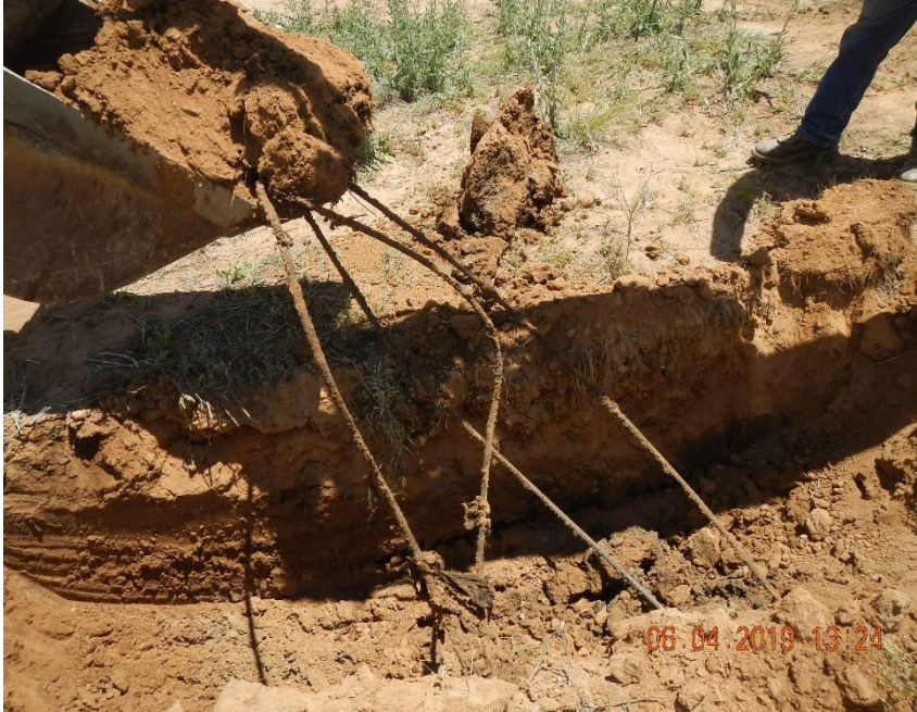
Wire rope and other debris found buried in trench #7.
