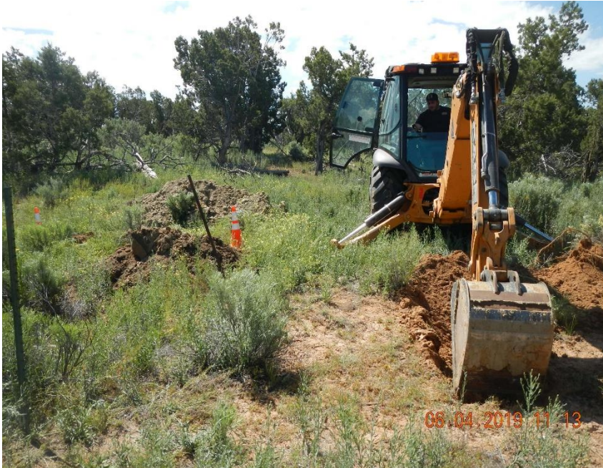
Excavating test trench along southwest side of pit.
