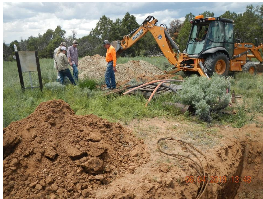
Additional test trenches dug to the west and southwest of the wellhead did not have visual impacts.
