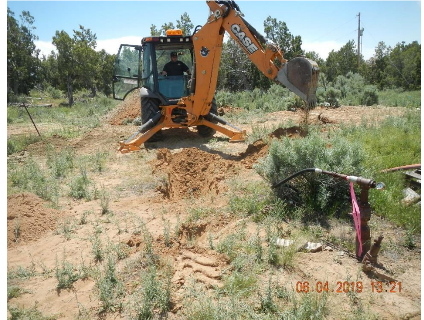
Beginning seventh test trench approximately 10' southeast of wellhead.
