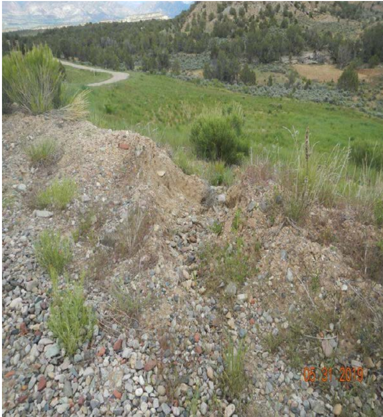
Photo#2: Washout at entry.
