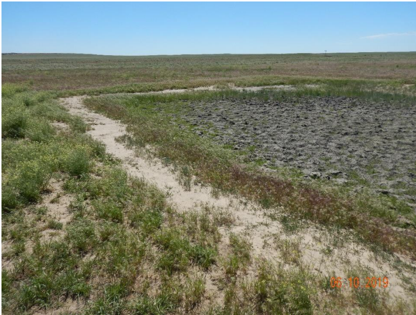
Photo 3: Photo taken from the north end of the pit, facing southeast. Photo shows pit has not been reclaimed. Photo also shows possible salt issues at the pit wall
