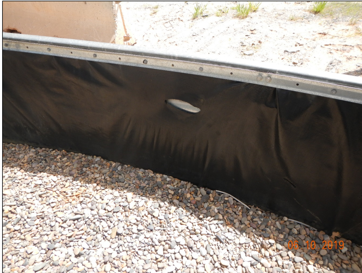
Photo #4 Holes in Tank liner.
