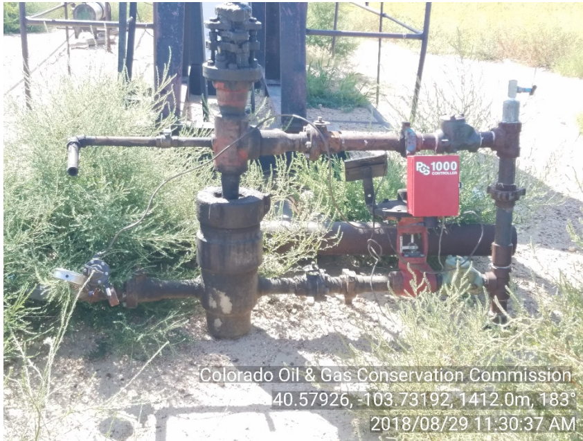
Photo #1 Chinook #1 (05-123-22590) Wellhead Shut-In | SI Weeds Bradenhead NOT plumbed to surface from prior insp.
