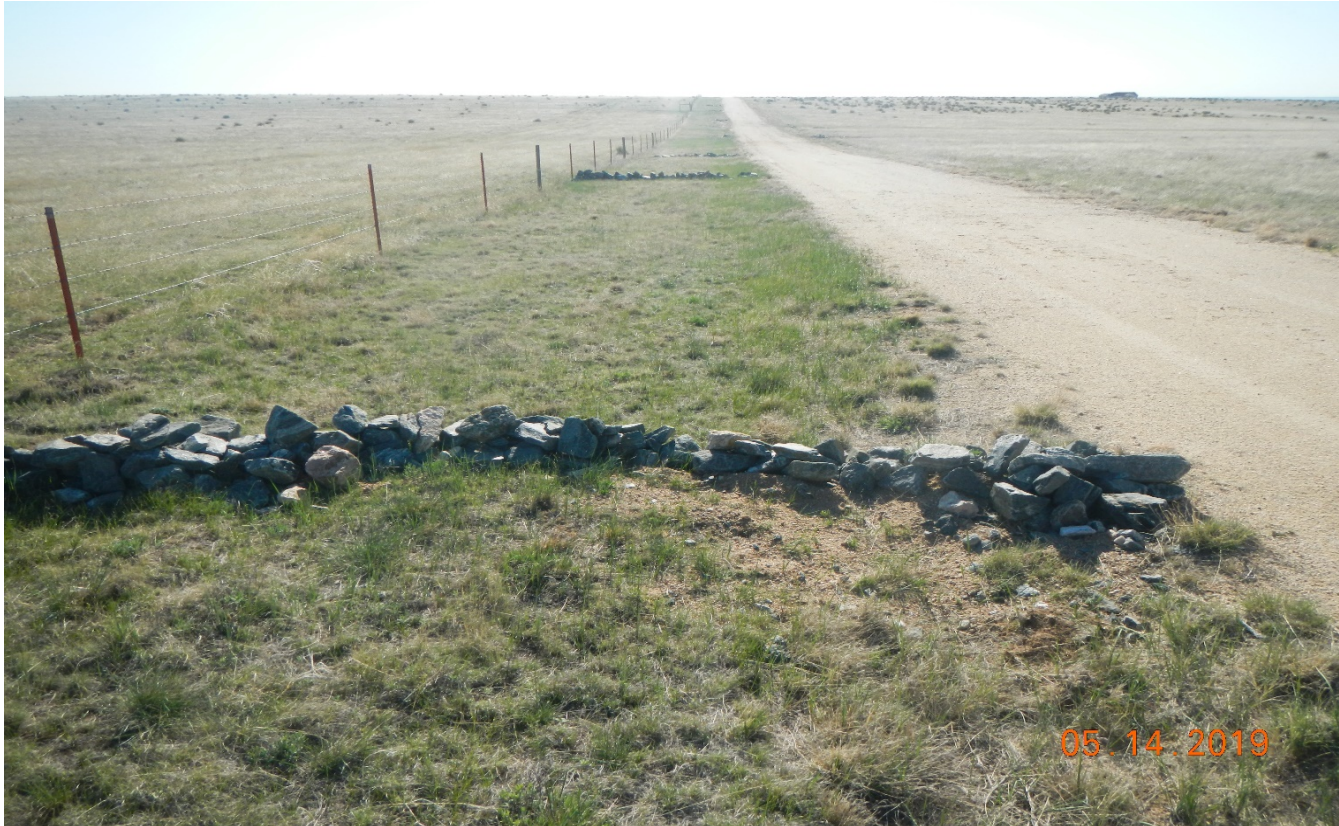
Photo 10. Rock check dams have been installed along the side of the road up gradient from the culverts. This photo depicts compliance of the corrective action.
