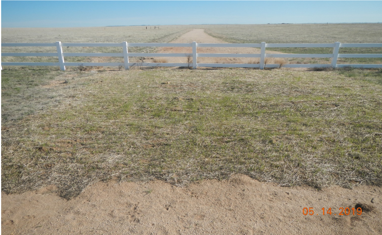
Photo 6. Facing north toward the access road. The side of the road was stabilized with straw blanket and vegetation is establishing. This photo depicts compliance of the corrective action.
