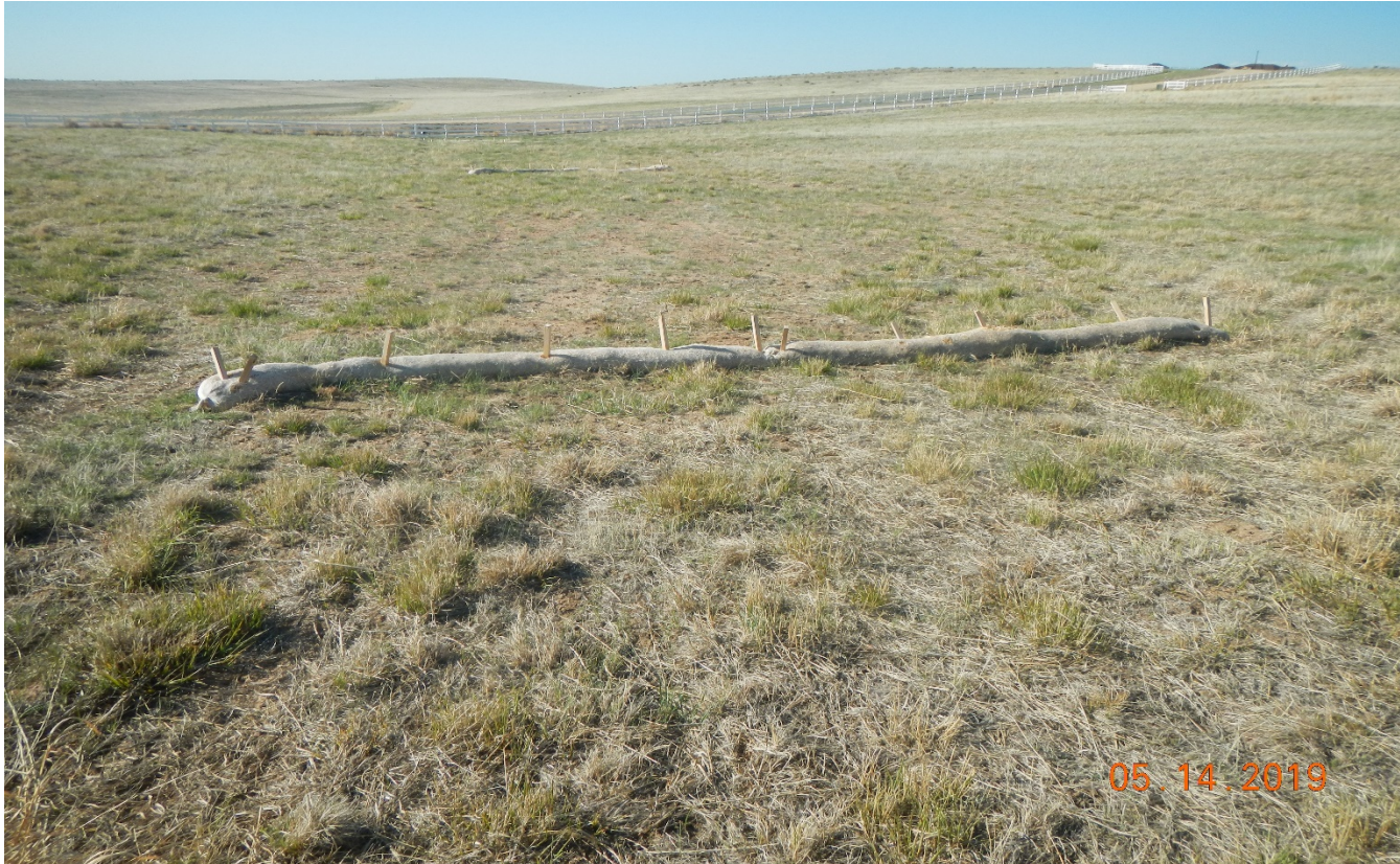
Photo 13. Facing south at the location. Wattles are installed at the bottom of the location. This photo depicts compliance of the corrective action.
