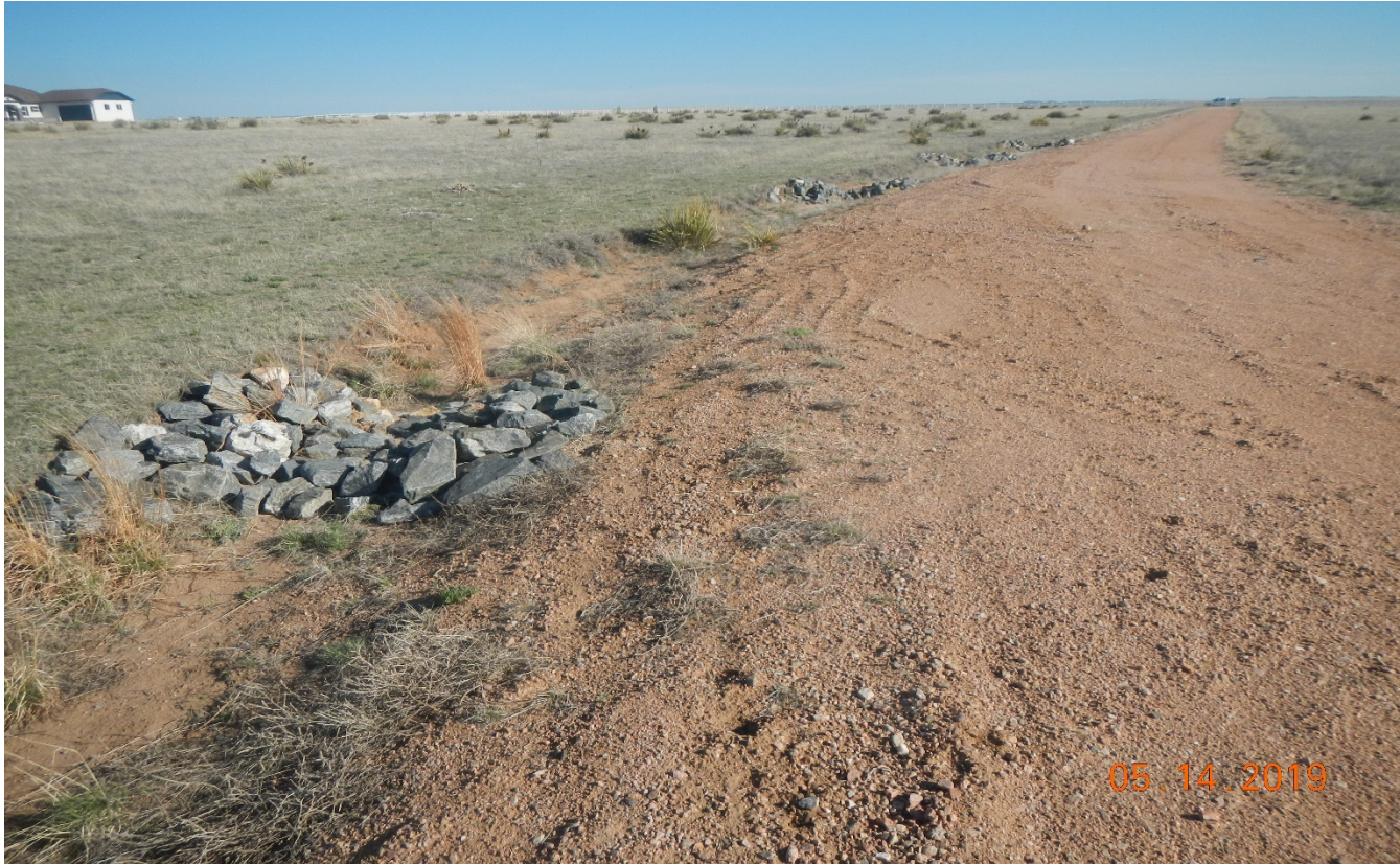
Photo 5. Rock check dams have been installed further up the road from the gate shown in photo 4. This photo depicts compliance of the corrective action.
