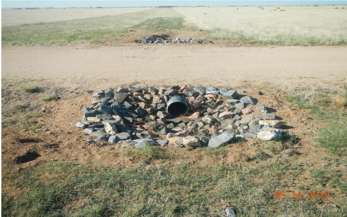
Photo 7. The inlet culvert rock rip/rap has been lowered to allow sediment to settle and not restrict stormwater flow. This photo depicts compliance of the corrective action.
