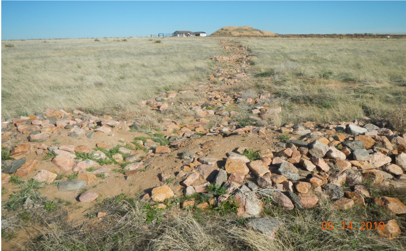
Photo 3. Standing out in the pasture facing northwest toward the road. The erosion channel has not been reclaimed and there is rock rip/rap scattered along the channel. This photo depicts noncompliance of the corrective action.
