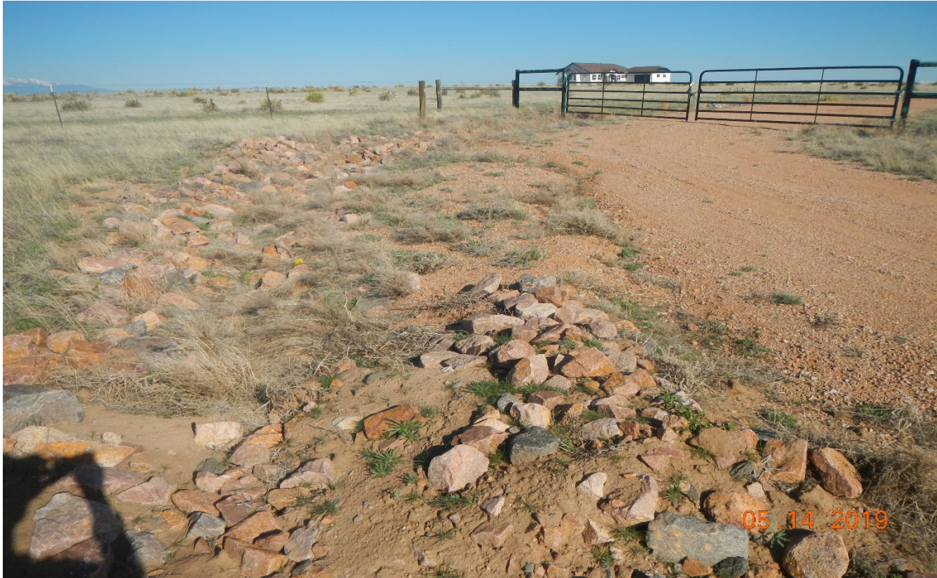
Photo 4. Rock rip/rap can be seen in the drainage channel. Rock check dams have been lowered to allow water flow. Weed debris has been removed from the channel. This photo depicts compliance of the corrective action.
