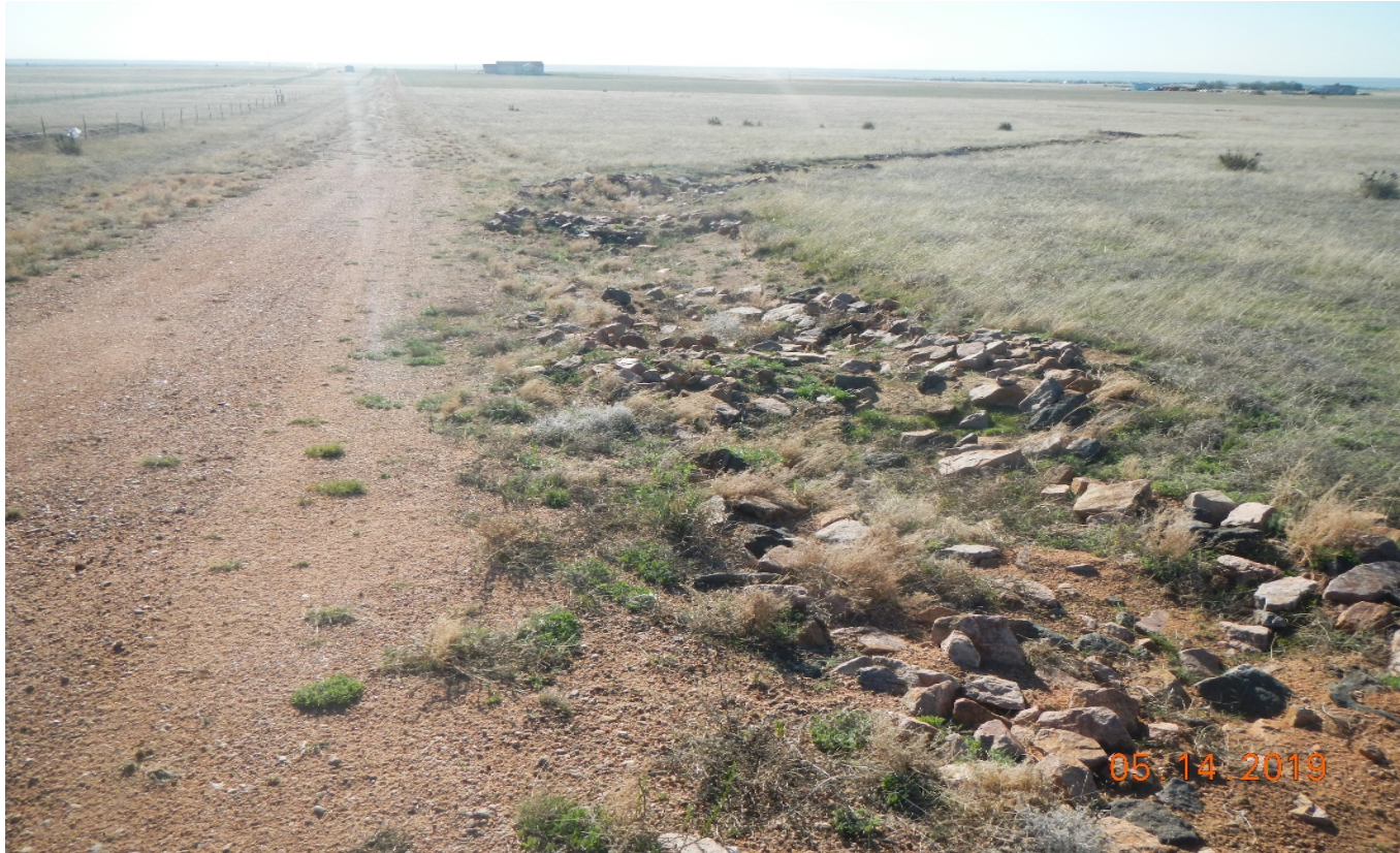
Photo 1. Facing east on the access road. Rock rip/rap can be seen in the drainage channel. Rock check dams have been lowered to allow water flow per previous inspection.
