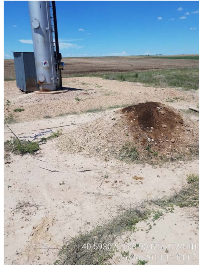
Photo 4 – Oily soil stockpiled on location.
