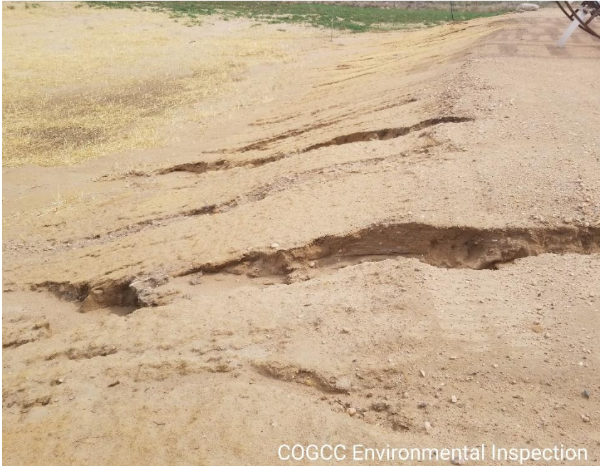
Photo 5 – Stormwater erosion caused by heavy storms have damaged hydromulch and other BMP's throughout facility. Spoke with operator and issues were identified prior to COGCC inspection. Repairs pending.
