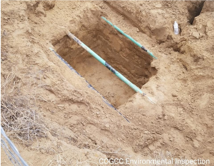
Photo 1 – Pipeline has been exposed via hydrovac and is awaiting spill cleanup.
