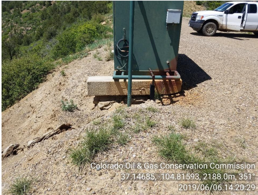
PHOTO 3: EROSION THAT APPEARS TO BE CAUSED FROM DRAINING THE SEPARATOR IN THE METER HOUSE AS THE METER HOUSE IS UPGRADE FROM LOCATION AND STORM WATER WOULD TRAVEL AWAY FROM THE METER HOUSE TOWARD THE CENTER OF LOCATION IS UNDERMINING METERHOUSE. REPAIR EROSION AND DISCONTINUE DRAINING SEPARATOR IN LOCATION. CA DATE 7/6/19
