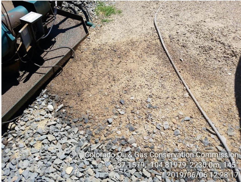
PHOTO 3: AREA OF IMPACTED SOIL APP. 7' BY 3' BETWEEN COMPRESSOR SKID AND PUMPJACK. Remove and dispose impacted material in approved manner, service and maintain equipment and self inspect to prevent recurrence of conditions per 1002.f(2) and 907. CA DATE 7/6/19.
