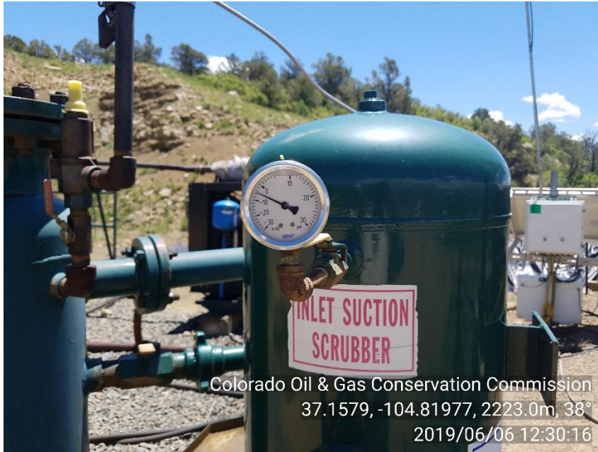
PHOTO 5: Vacuum pump observed on well without COGCC approval. Provide COGCC with documentation showing approval of use of vacuum pump. CA DATE 6/21/19.
