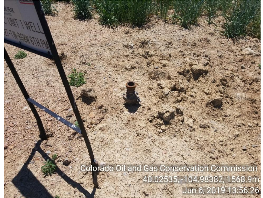
Photo 2 WH appears to be removed. Flow line has not been removed.
