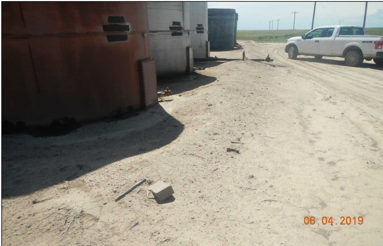
Photo 6. The berm around the north side of the tanks is insufficient for secondary containment.
