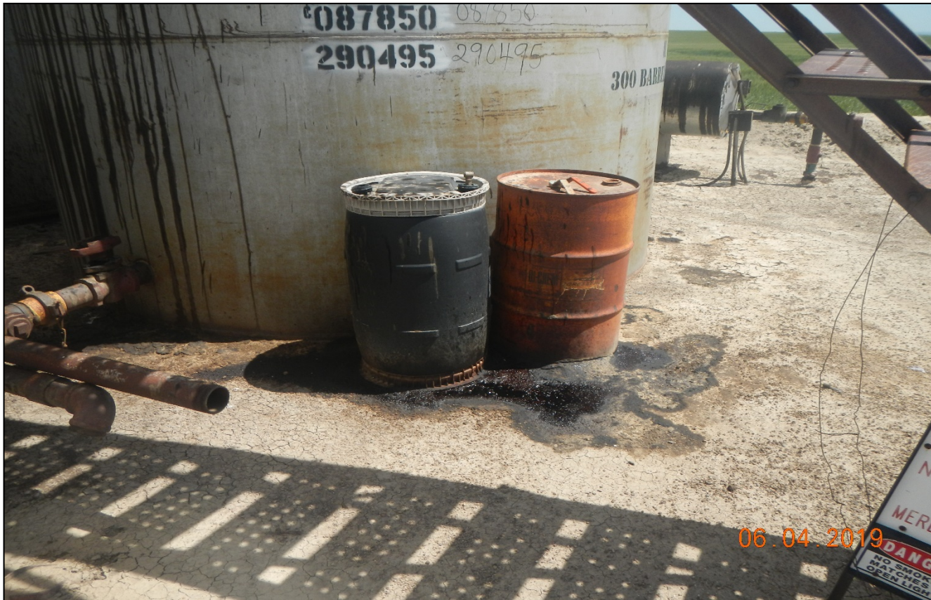
Photo 2. There are two barrels with no labeling and possible leakage with oil stained soil.
