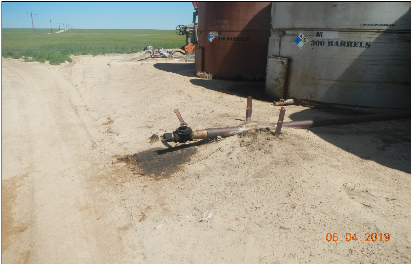
Photo 4. There is oil stain soil at the pipe valve.
