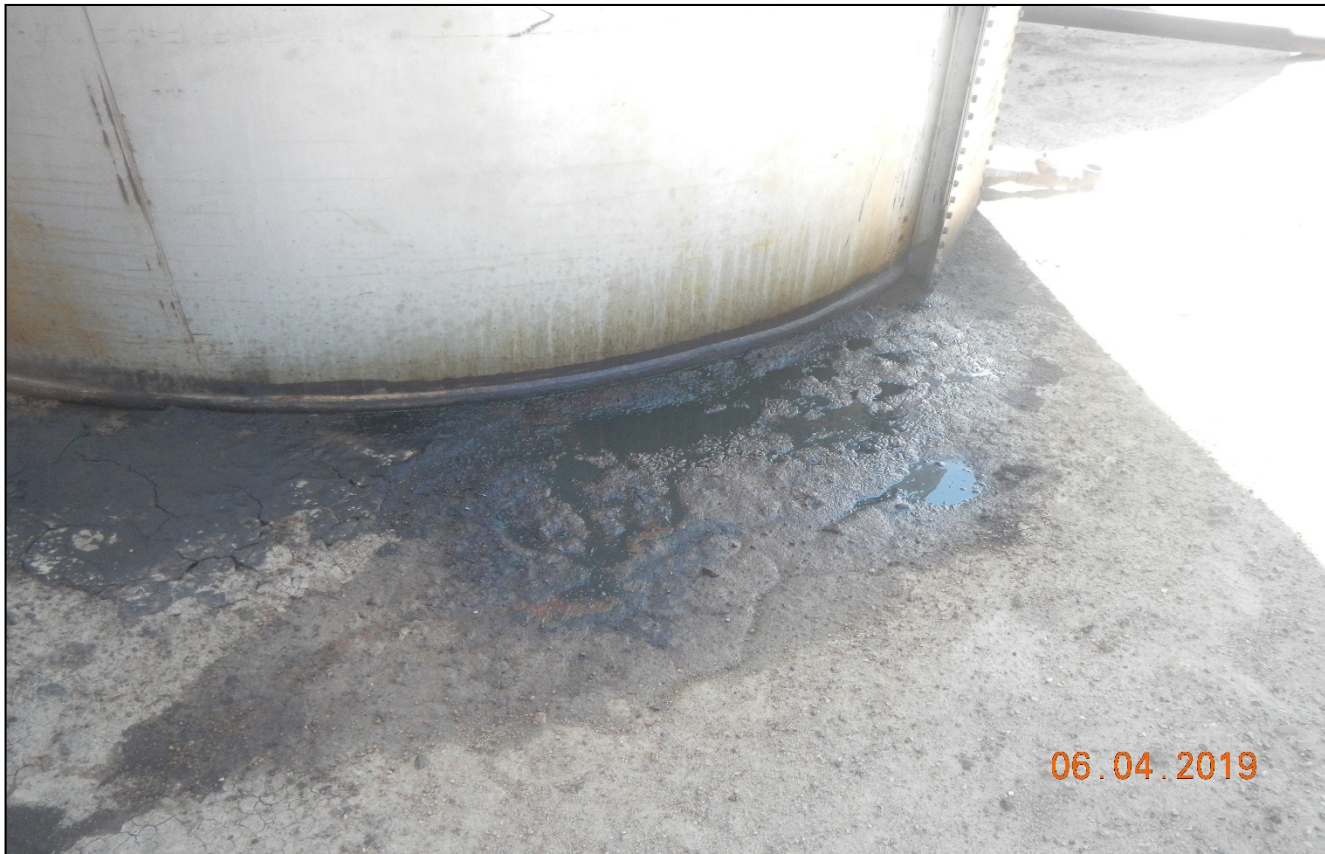
Photo 5. There is oil stained soil around the tank. Tank likely has leak.
