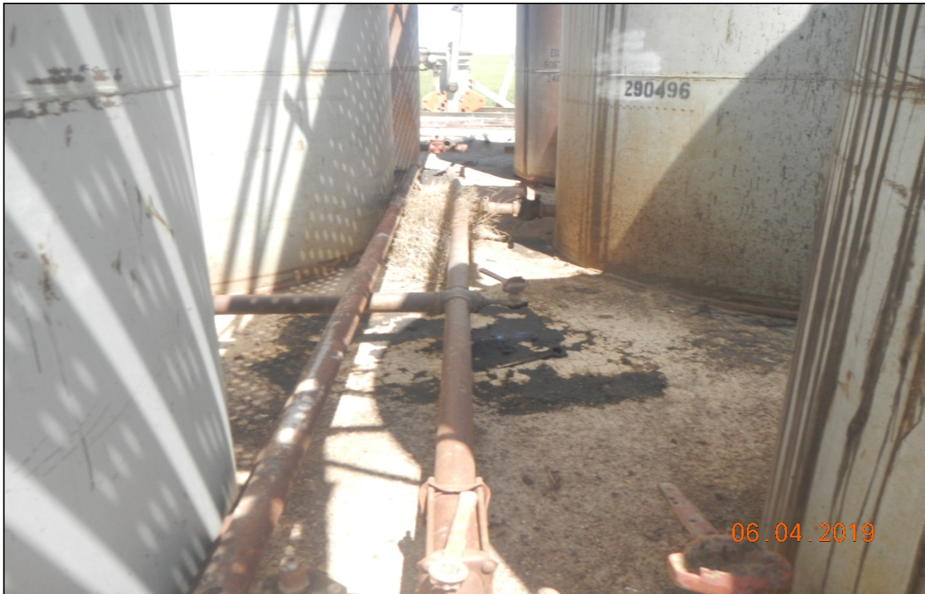
Photo 3. There is oil stained soil between the tanks.
