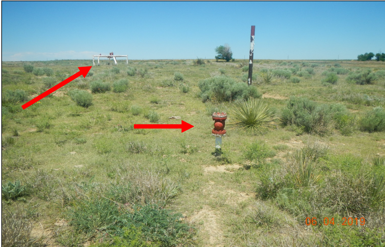
Photo 7. There is a single pipe riser that remains at the north side of location. Another riser further north may be an active line per previous inspection.
