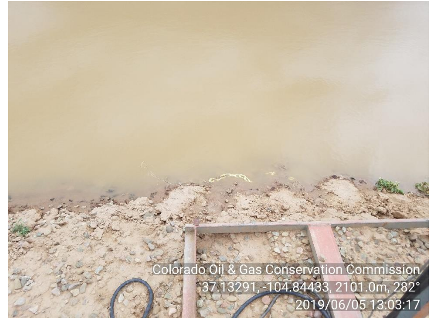
PHOTO 8: PRODUCED WATER IS ABOVE FREEPOINT MARKER. SPOKE WITH JACK WISEMAN WITH EVERGREEN TO HAVE PIT DRAINED. WATER TRUCKS ARRIVED ON LOCATION WHILE I WAS STILL INSPECTING AND DRAINED THE PIT. Lower fluid level so at least two feet of freeboard exists per Rule 902.b. CA DATE 6/6/19.
