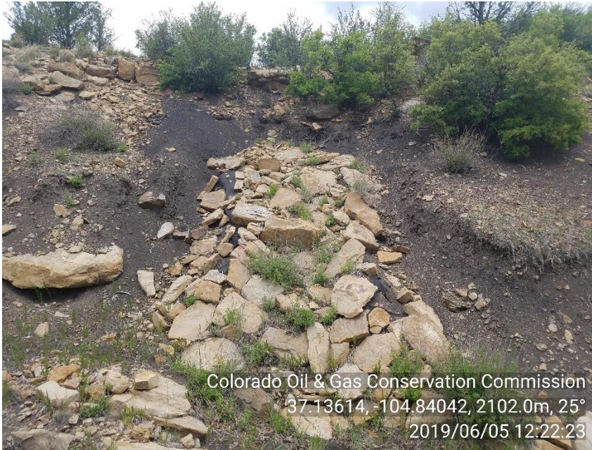
PHOTO 7: STORMWATER IS BYPASSING BMP'S INSTALLED ON ROW HILLSIDE CUT. REPAIR EROSION AND INSTALL BMP'S TO ENSURE STORMWATER CANNOT BYPASS EXISTING BMP'S IN ACCORDANCE WITH 1002 SERIES RULES. CA DATE 7/5/19
