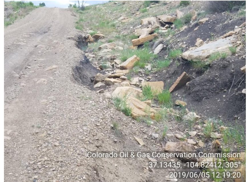
PHOTO 4: EROSION FURTHER UP GRADE FROM PREVIOUS PHOTO. EXSISTING BMP'S APPEAR TO HAVE FAILED. REPAIR EROSION AND REINSTALL BMP'S TO PREVENT FURTHER EROSION OF ROW IN ACCORDANCE WITH 1002 SERIES RULES. CA DATE 7/5/19.
