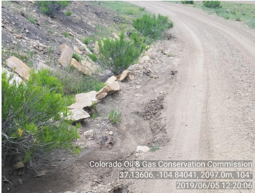
PHOTO 5: IMAGE OF POINT WHERE STORMWATER IS BYPASSING BMP'S NOTED IN PHOTO #3. REPAIR EROSION AND INSTALL BMP'S TO ENSURE STORMWATER CANNOT BYPASS EXISTING BMP'S IN ACCORDANCE WITH 1002 SERIES RULES. CA DATE 7/5/19
