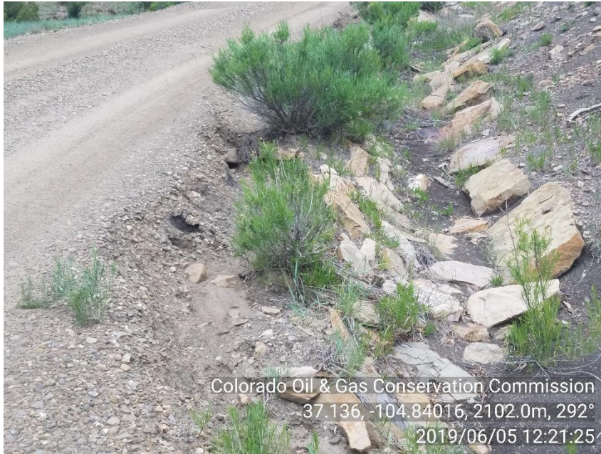
PHOTO 3: STORMWATER IS BYPASSING THE ROCK LINED DITCH AND ERODING THE LEASE ROAD WEST OF LOCATION ROW ENTRANCE ON THE MAIN ROAD. REPAIR EROSION AND INSTALL BMP'S TO ENSURE STORMWATER CANNOT BYPASS EXISTING BMP'S IN ACCORDANCE WITH 1002 SERIES RULES. CA DATE 7/5/19
