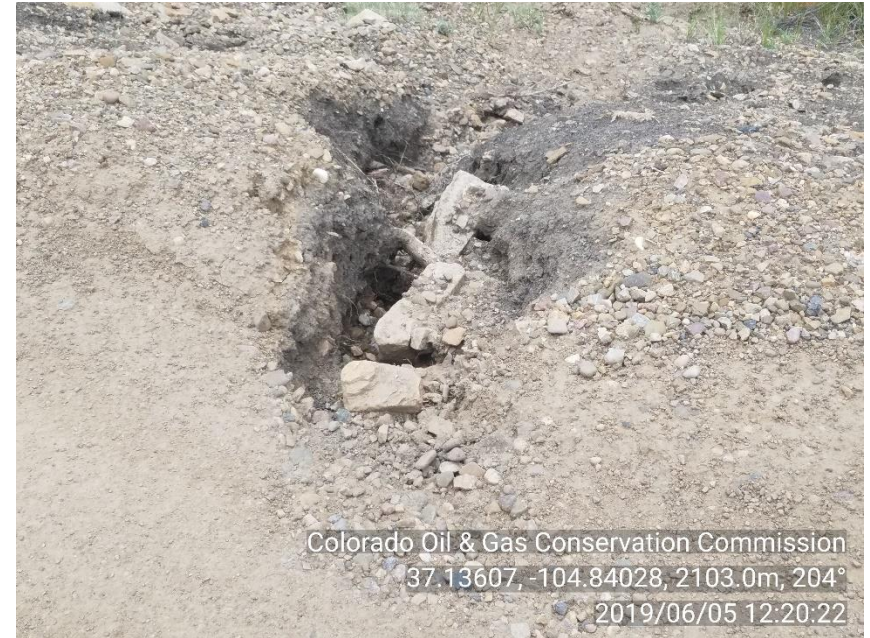
PHOTO 6: EROSION ON DOWN GRADE SIDE OF ROW ACROSS FROM EROSION ON PREVIOUS PHOTOS. REPAIR EROSION AND REINSTALL BMP'S TO PREVENT FURTHER EROSION OF ROW IN ACCORDANCE WITH 1002 SERIES RULES. CA DATE 7/5/19.
