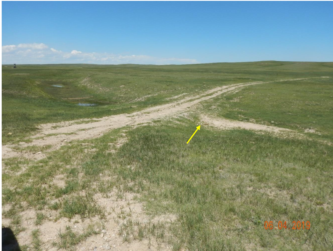
Photo 5: Photo taken from the access road, facing northwest. Photo shows section of access road that crosses a drainage. Photo shows erosion degradation and sediment transport off road. Access road remains and has not been reclaimed
