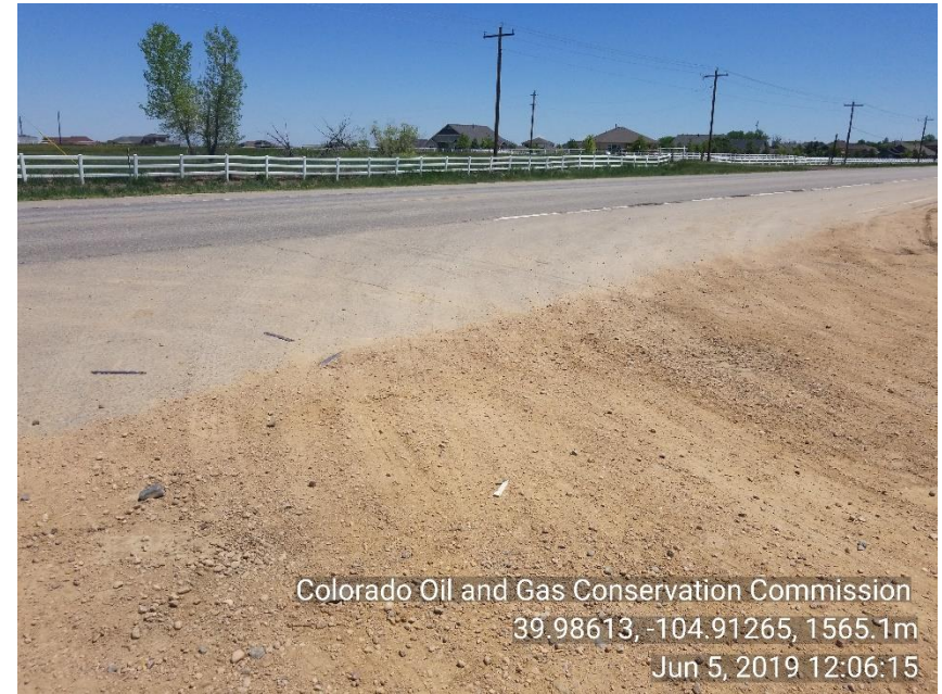
Photo 6 Sediment tracking onto HWY 7 from Monaco street
