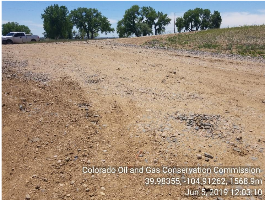
Photo 3 tracking pad to location impacted with sediment
