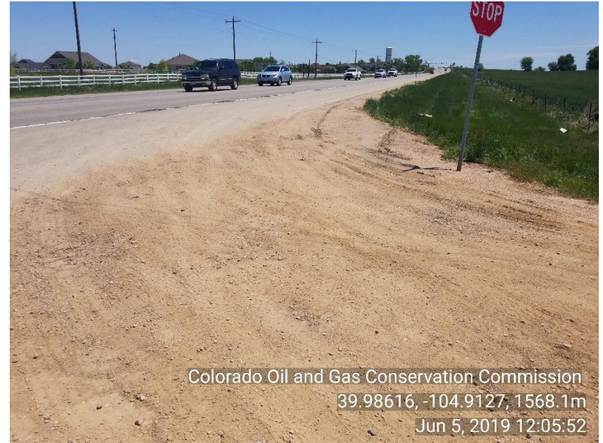
Photo 4 Sediment tracking onto HWY 7 from Monaco street
