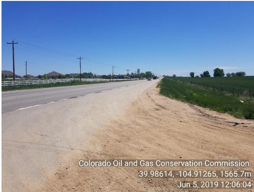
Photo 5 Sediment tracking onto HWY 7 from Monaco street
