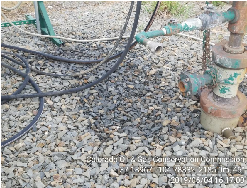
PHOTO 3: AREA OF IMPACTED GRAVEL AROUND WELLHEAD APP. 2' BY 4' IN SIZE. Remove and dispose impacted material in approved manner, service and maintain equipment and self inspect to prevent recurrence of conditions per 1002.f(2) and 907" CA DATE 7/4/19
