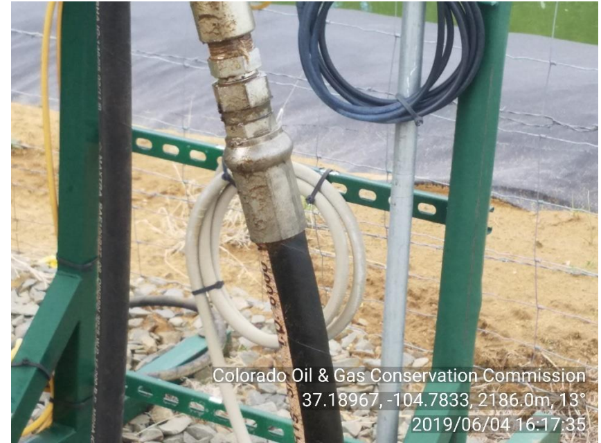
PHOTO 4: HYDRAULIC FITTING APPEARS TO BE SEEPING FLUID. Increase frequency of maintenance and self inspection schedule of equipment to prevent impacting surface materials and mixing of wastes with precipitation" CA DATE 7/4/19
