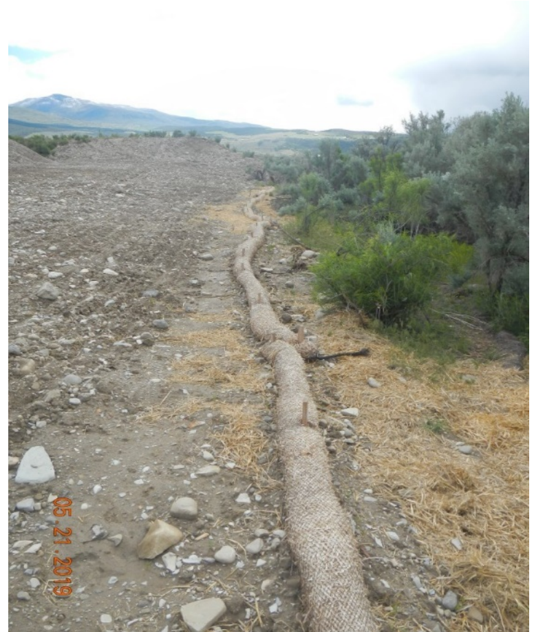
Photo#4: Wattles installed as perimeter controls.
