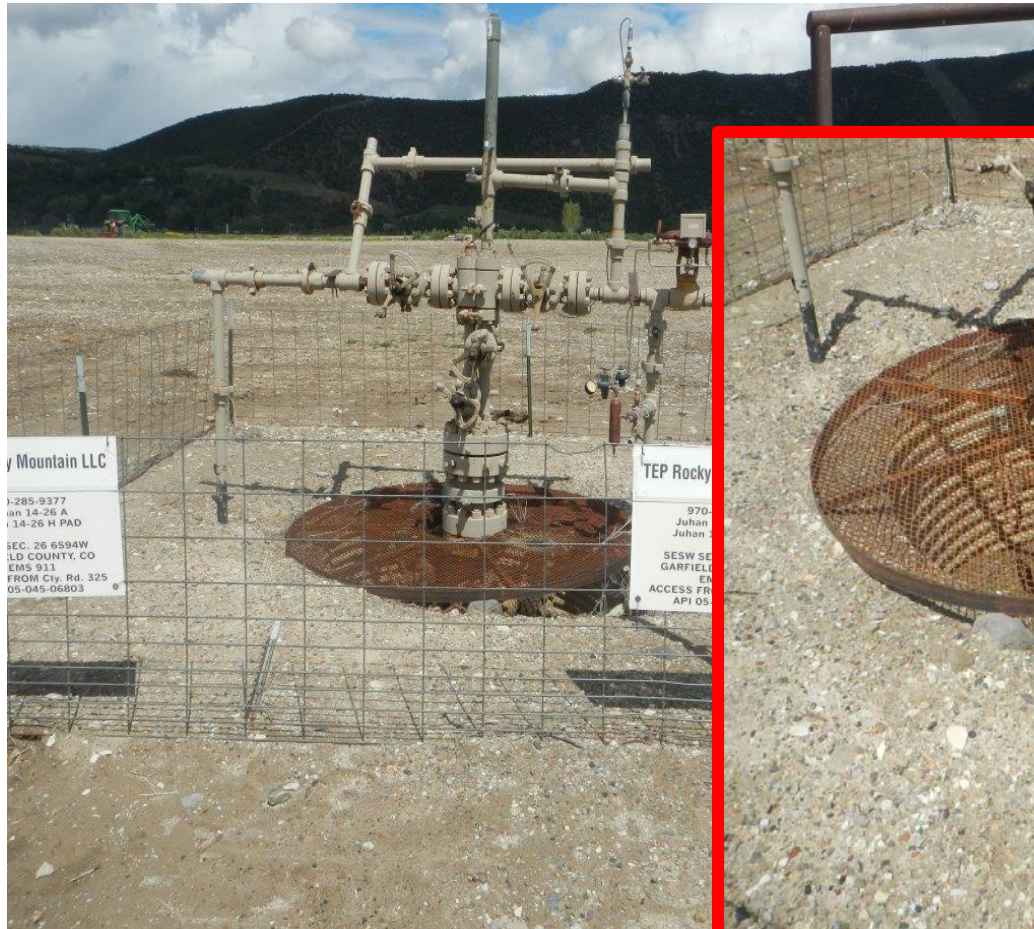
Photo#5: Cellar grate (cover) has a gap on Southeast side.
