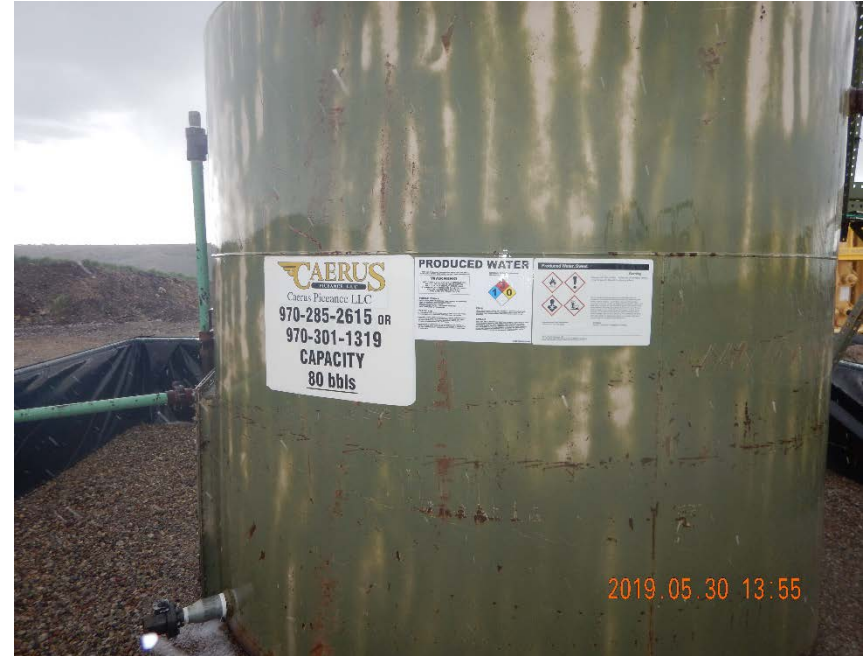
Photo #6 – Close up on 80 bbl produced water AST.
