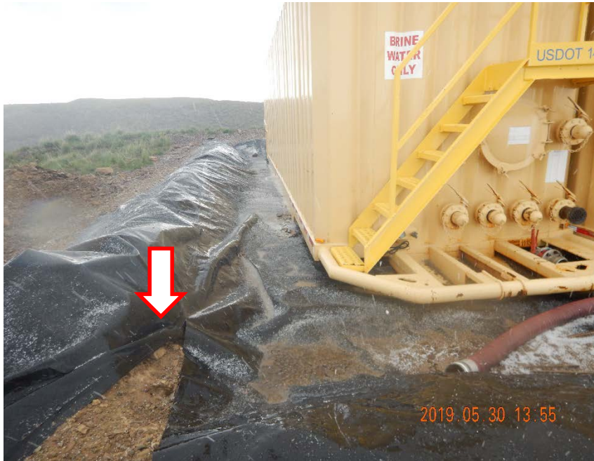
Photo #7 – View of parted liner in NW corner of frac tank battery. Note storage of hose with metal fitting in contact with battery liner.
