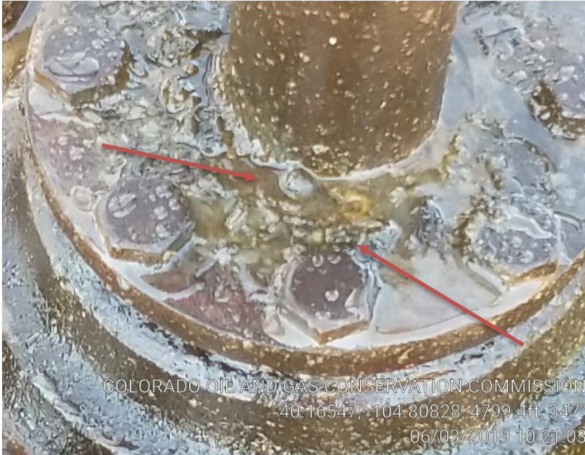
Pic 5 bubbles on wellhead
