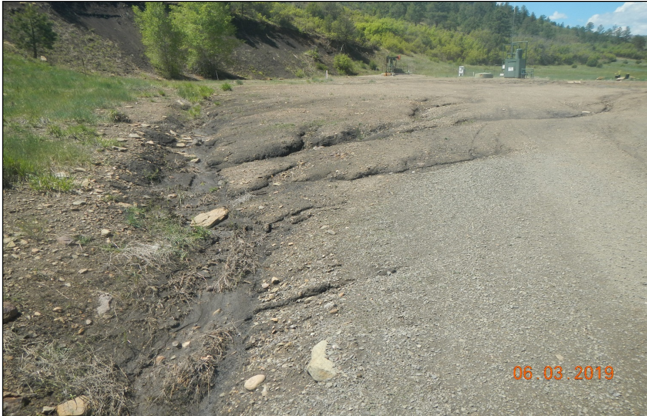
Photo 2. Facing southwest toward the location. There are erosion issues coming off the pad surface and is depositing sediment into the culvert along the access road.
