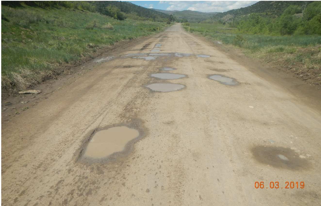
Photo 1. The main southfork road has areas of road damage that needs to be graded.
