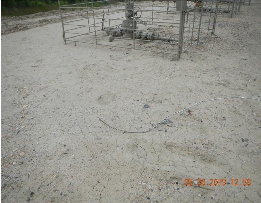
Unused buried 1/2" tubing ran from separator to well 23-4D
