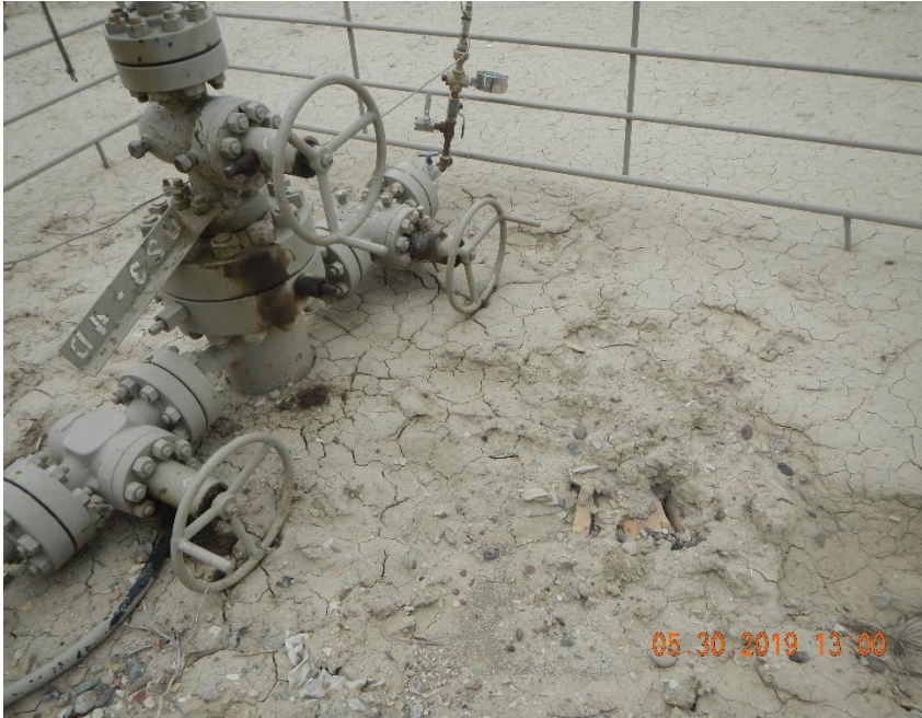
Rathole has subsided and is exposed.
