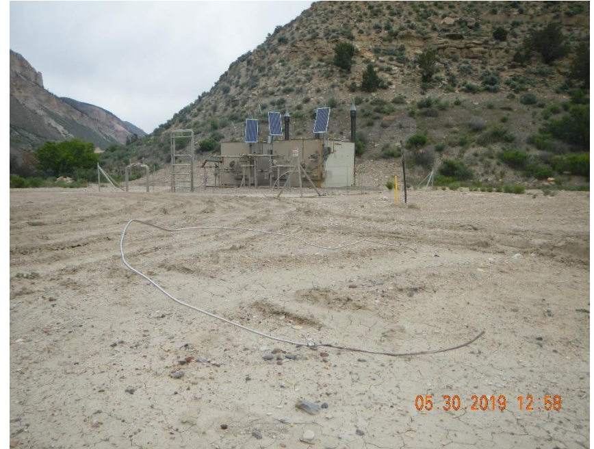
Unused buried 1/2" tubing ran from separator to well 23-4D
