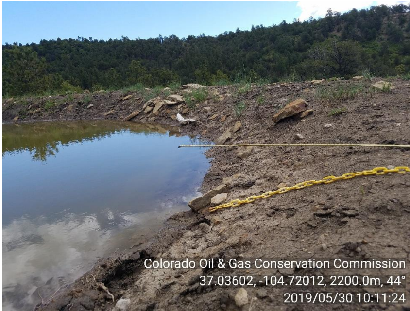
PHOTO 3: PRODUCED WATER LEVEL IS ABOVE 2' FREEBOARD. CONTACTED JACK WISEMAN WITH EVERGREEN TO HAVE PIT DRAINED TO MAINTAIN 2' FREEBOARD. Lower fluid level so at least two feet of freeboard exists per Rule 902.b. CA DATE 5/31/19.
