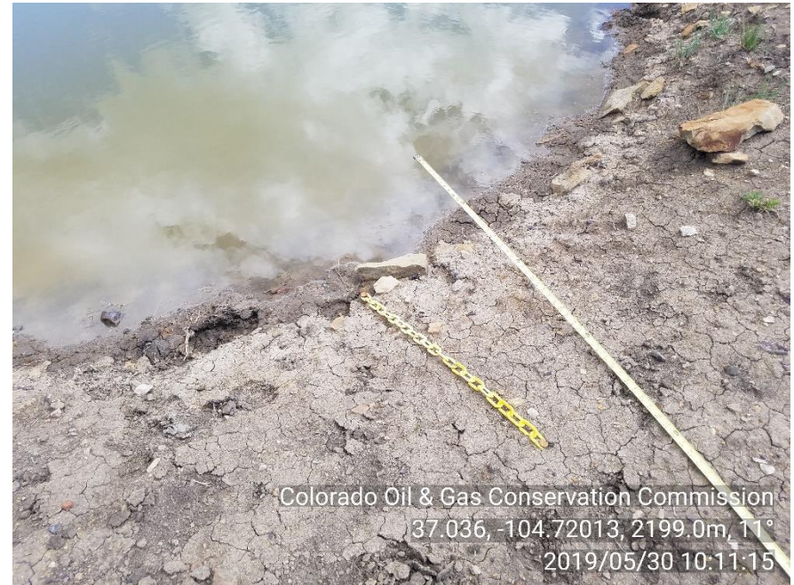
PHOTO 4: FREEBOARD MARKER IS INCORRECTLY INSTALLED AND IS NOT DEPICTING A 2' VERTICAL DEPTH FROM THE LOWEST PIT BERM ELEVATION. INSTALL FREEBOARD MARKER IN ACCORDANCE WITH 902 SERIES RULES. CA DATE 5/31/19.
