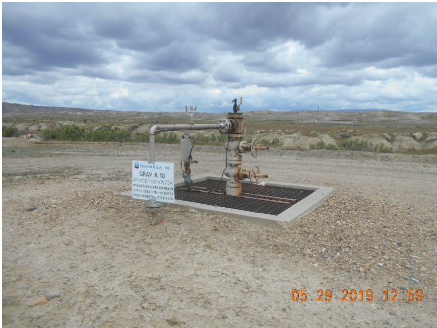
Injection wellhead
