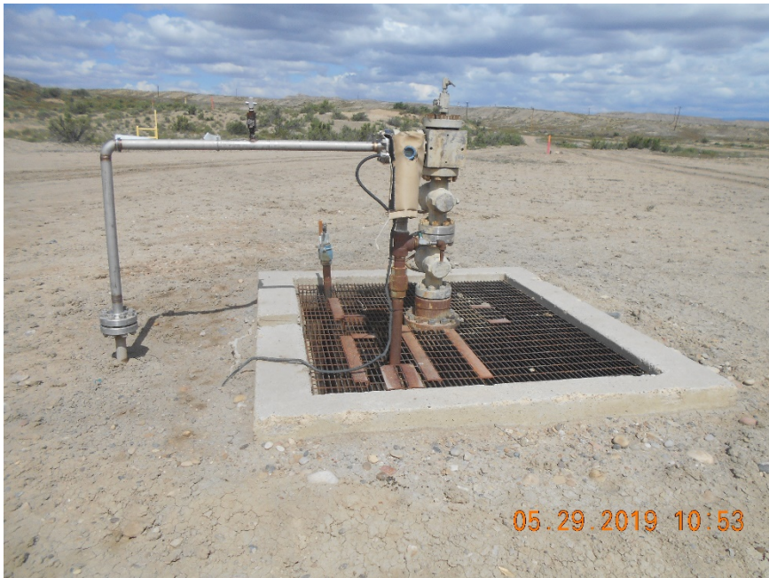
Injection wellhead
