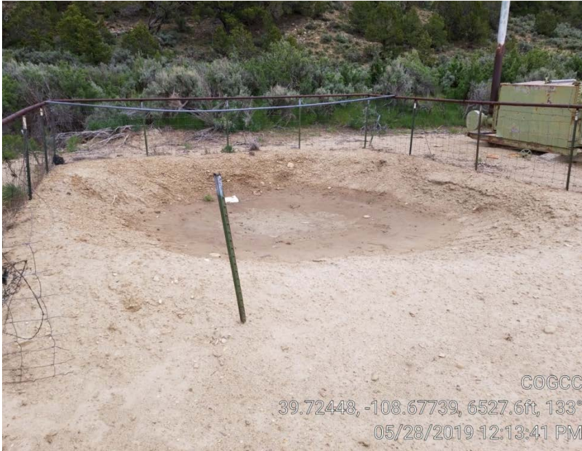
Photo 2. Pit without fence on one side.
