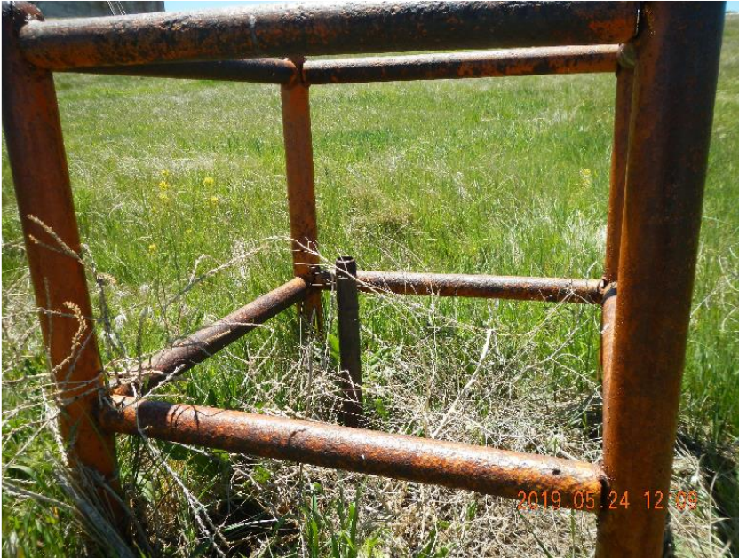
Photo 13: 1" riser inside barrier.
