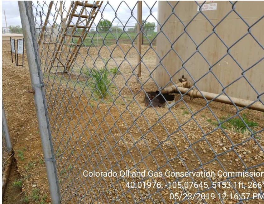
Photo 5 – Eroding berm surrounding tank battery near loadout
