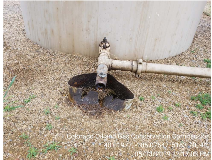
Photo 6 – Stained oil at loadout
