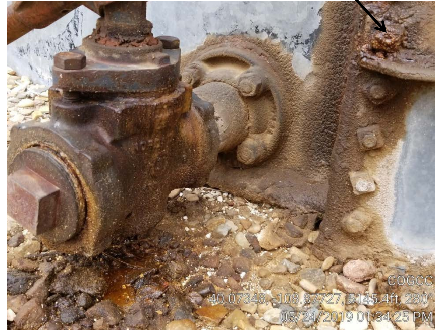
Photo 4. Fluid seeping at bolt.
