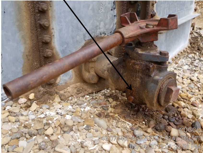
Photo 3. Valve leaking fluid at ~1 drop every 4 seconds.
