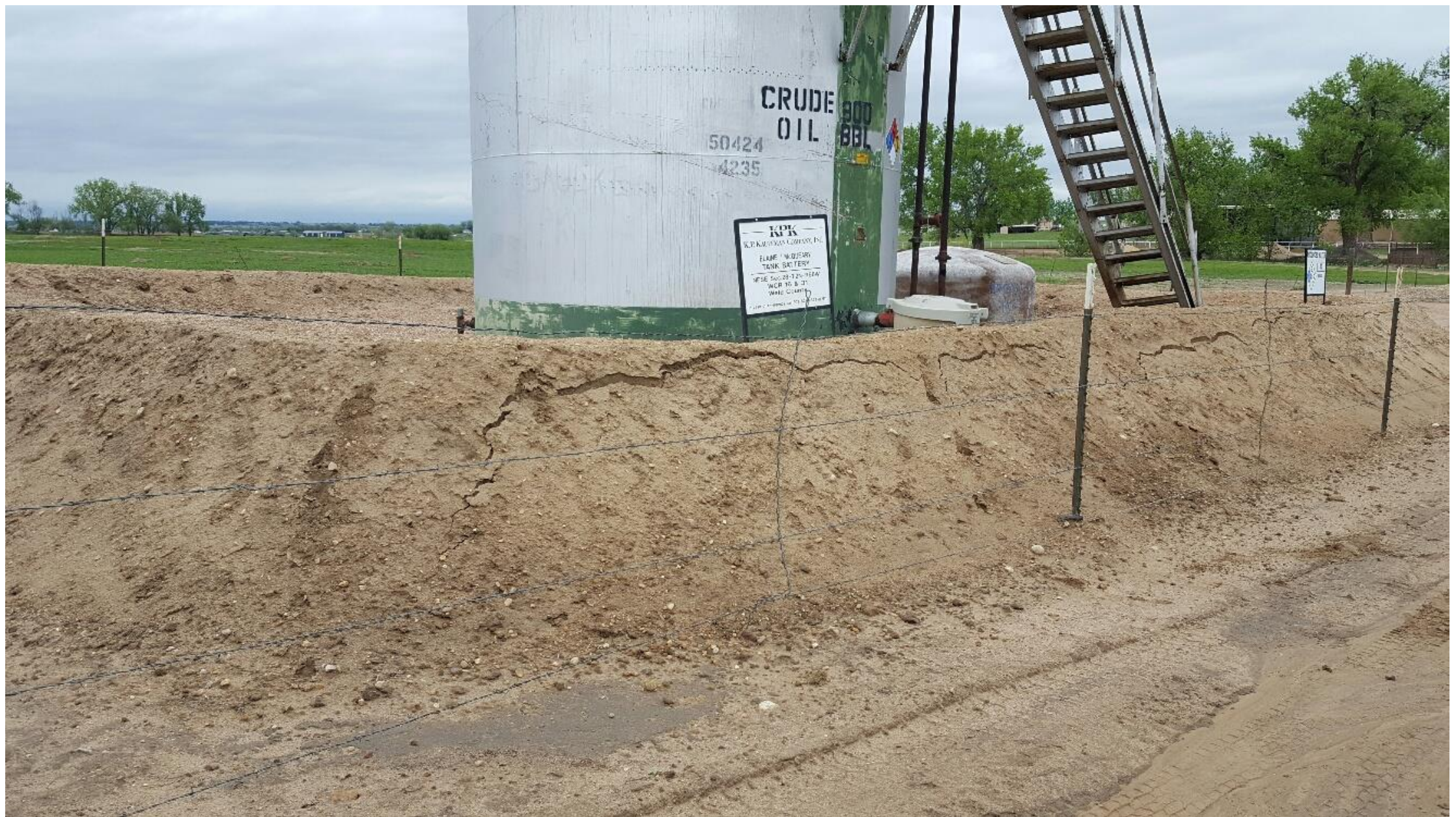
Figure #2 Berms have been repaired.
